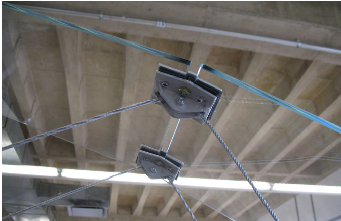
Figure 16: Glass "clamp" detail
