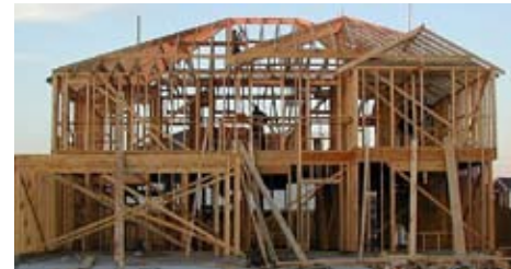
Fig. 4. Stick & Frame Construction
