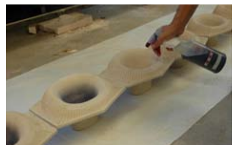
Fig. 110. application of mason stain
