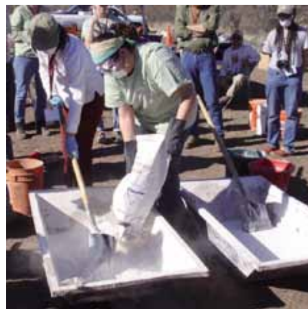
Figure 6: INAH restoration architect Abby Valenzuela Rivera demonstrating lime slaking - the hydration process in the production of lime plaster - as part of TICRAT 2013.
