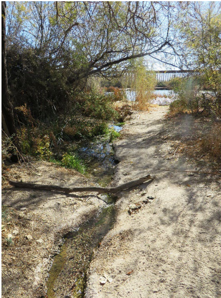
Figure 3-38 Concrete-lined spring outflow stream channel (Nov. 2022). Teresa DeKoker, photographer
