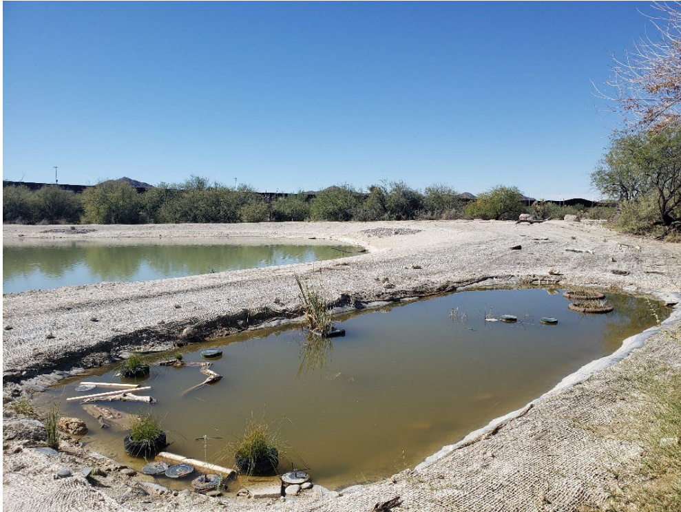
Figure 5-6 Sediment trap pool constructed in Spring 2022 (Nov. 2022). Teresa DeKoker, photographer
