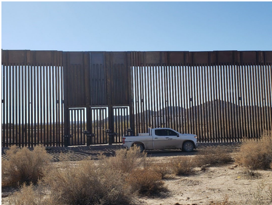
Figure 5-17 Border infrastructure road (Nov. 2021). Teresa DeKoker, photographer
