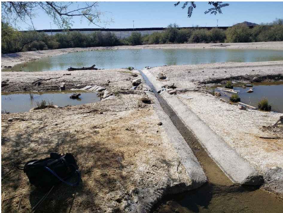
Figure 5-15 Straight portion of concrete channel (Nov. 2022). Teresa DeKoker, photographer
