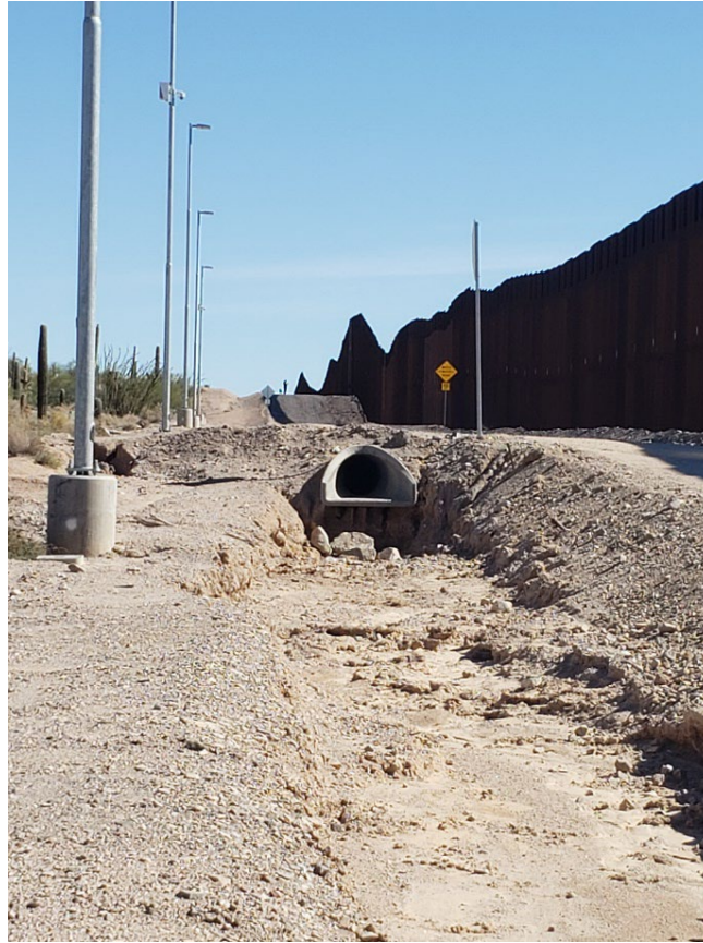
Figure 5-18 Border infrastructure road and drainage ditch (Nov. 2022). Teresa DeKoker, photographer
