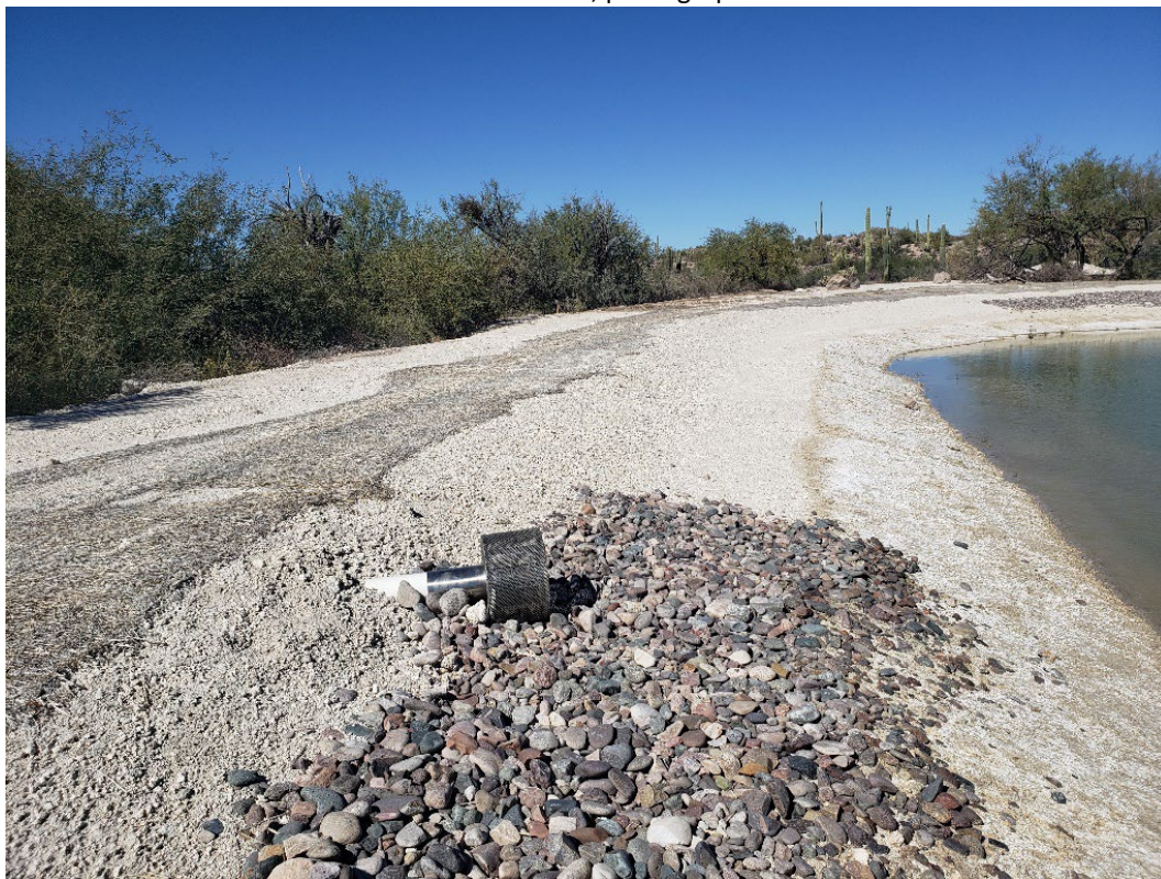
Figure 3-50 Berm on west end of pond facing north with outflow pipe post restoration (Nov. 2022). Teresa DeKoker, photographer
