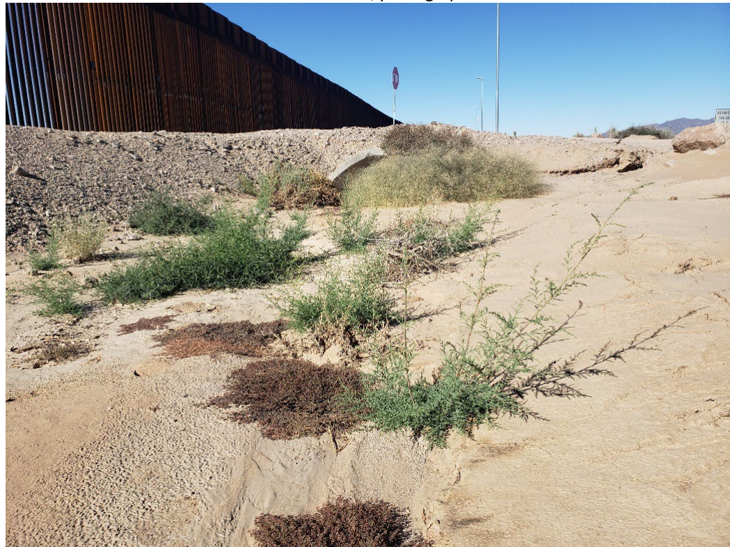
Figure 3-52 Drainage ditch with tamarisk growing, facing west (Nov. 2022). Teresa DeKoker, photographer
