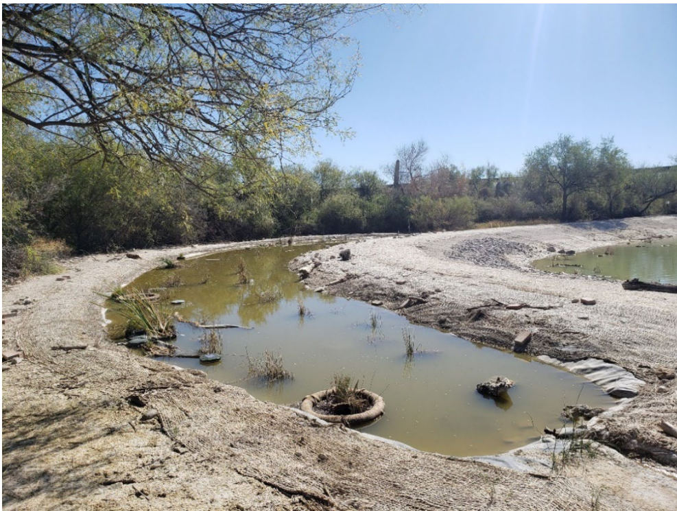
Figure 5-5 Newly constructed sediment trap pool (Nov. 2022). Teresa DeKoker, photographer
