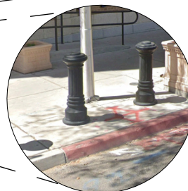
The sidewalk provides safety to pedestrians by placing safety poles around acting as a barrier to reduce any pedestrian and motor vehicle accidents.
