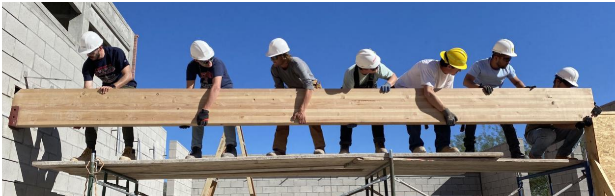
Figure 4. Students install a glue-laminated beam at a design build project.
