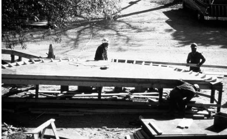
5. Carpenters preparing formwork for cycloid shells. Forth Worth, 1969.
