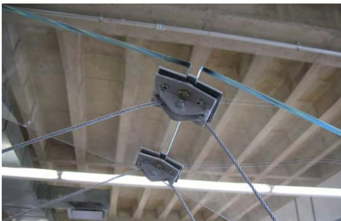
Figure 16: Glass "clamp" detail
