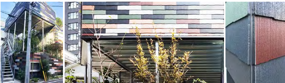
Figure 13: Context Coloring Siding, Overlap House, Tokyo, Japan, Akihisa Hirata Architecture Office (2019)
