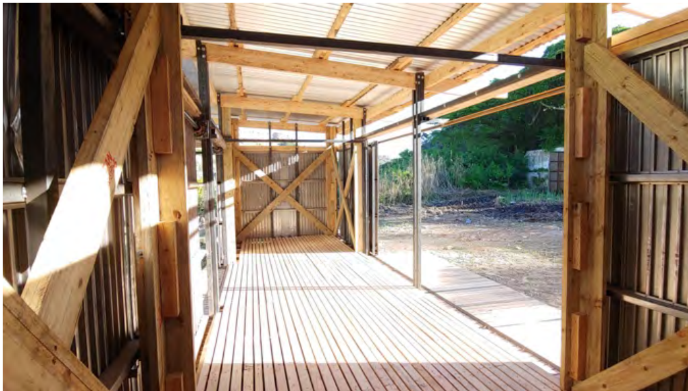
Figure 4: Laminated wood scrap for the roof structure reserved more valued materials for other structures and uses (Shall 2019).
