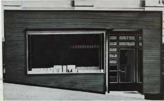
Figure 4 All Metal Store Front in Lausanne, Switzerland. Source: The Kawneer Book of Store Fronts, 1936.
