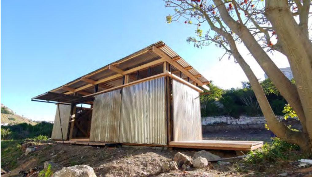
Figure 2: The community event- and maker-space was constructed of scavenged materials using common tools and accessible means. The final work was completed in less than 10 days with a team of 11 for under $1500 (Shall 2019).
