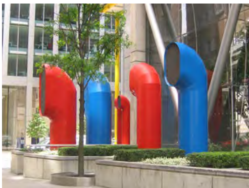
Figure 3: Ventilation fixtures at 88 Wood Street by The Richard Rogers Partnership, constructed 1994-98. Source: (Ford 2008).
