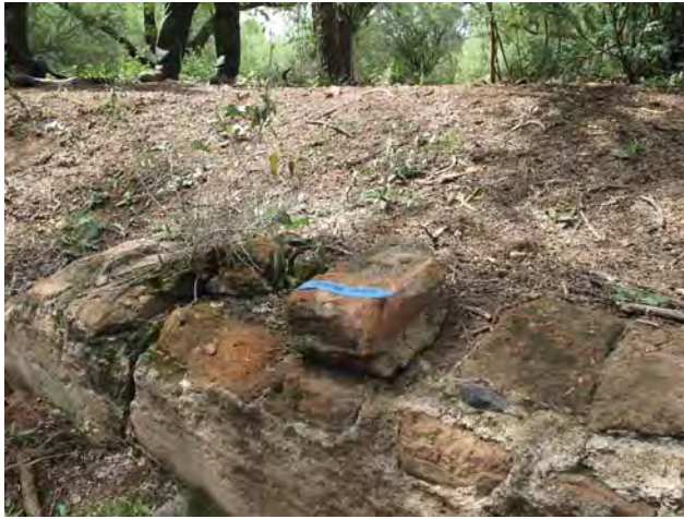
Figure 4: Photo of loose brick and plaster sample prior to removal.
