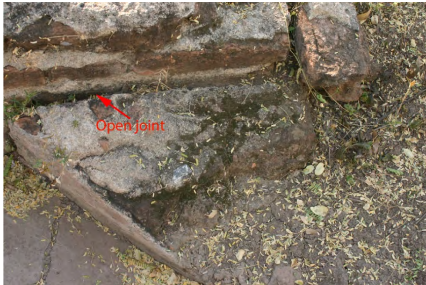
Figure 3.13. Detail of open joint between the west wall of the compuerta and the west half of the weir at the northern end of the feature. Note vegetation encroachment within gap (photographed November 19, 2013).
