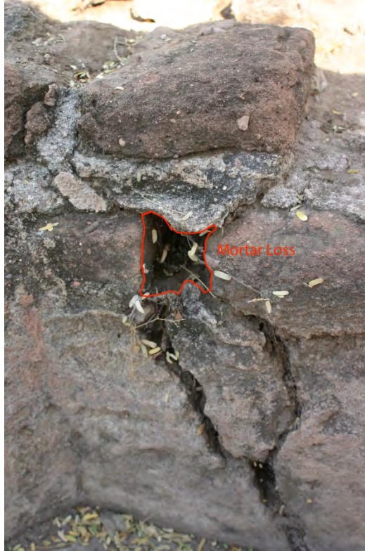
Figure 3.20. North end of east compuerta wall showing mortar loss within brick joints, outlined in red (photograph facing northeast, November 19, 2013).
