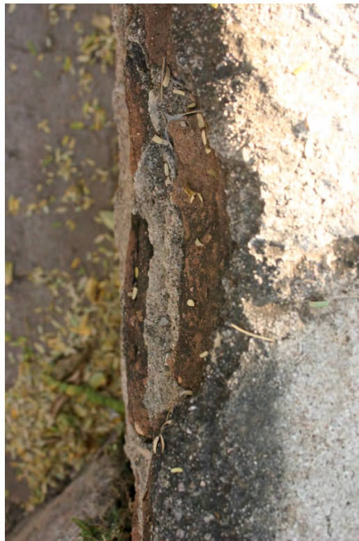
Figure 3.17. Plan view of spalled brick, showing extent of material loss (photographed November 19, 2013).
