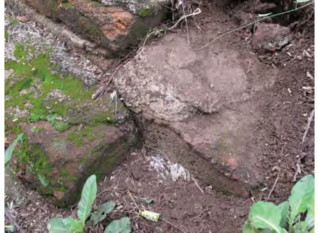
Figure 7: Photo of exposed bedding mortar after removing the brick above.
