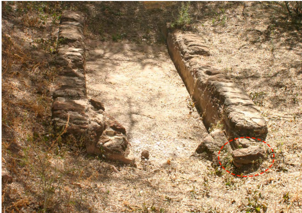
Figure 3.24. Loose brick at northwest corner of compuerta, outlined in red (photograph facing southeast, November 19, 2013).
