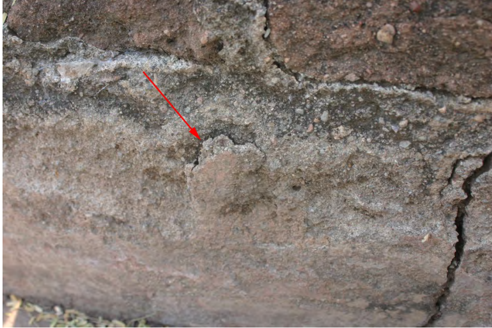
Figure 3.23. Spalling plaster near center of the east compuerta wall (photograph facing east, November 19, 2013).
