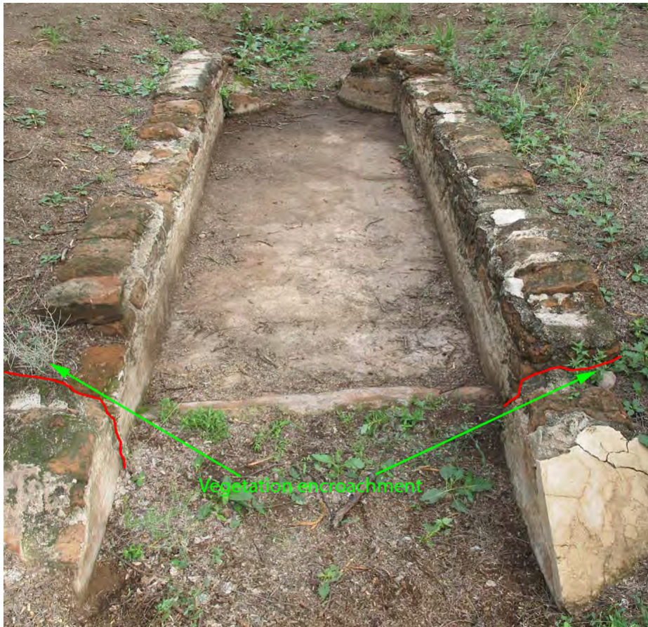
Figure 3.10. Structural cracks in southern ends of both east and west compuerta walls (traced in red); note vegetation encroachment in cracks (see detail in Figure 3.9) (photographed November 19, 2013).
