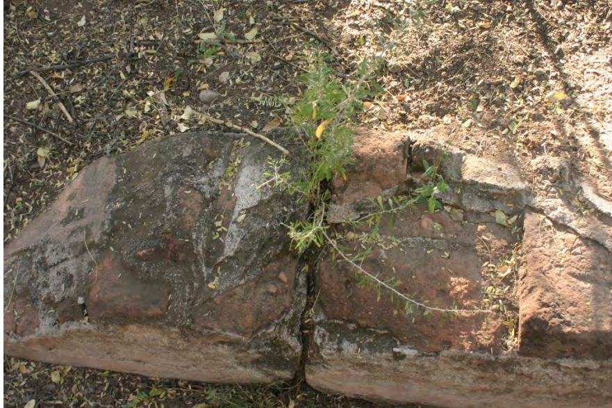
Figure 3.11. Structural crack in southern end of west wall; vegetation encroachment within crack (photographed November 19, 2014).
