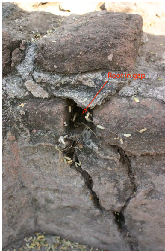
Figure 3.12. Structural crack in north east corner of compuerta. Note root in the gap of the bedding mortar (photographed November 19, 2014).
