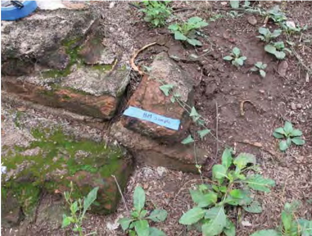
Figure 6: Photo of compuerta wall prior to removing the bedding mortar sample.
