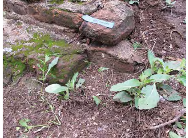
Figure 9: Photo of the compuerta wall after the mortar sample was removed.
