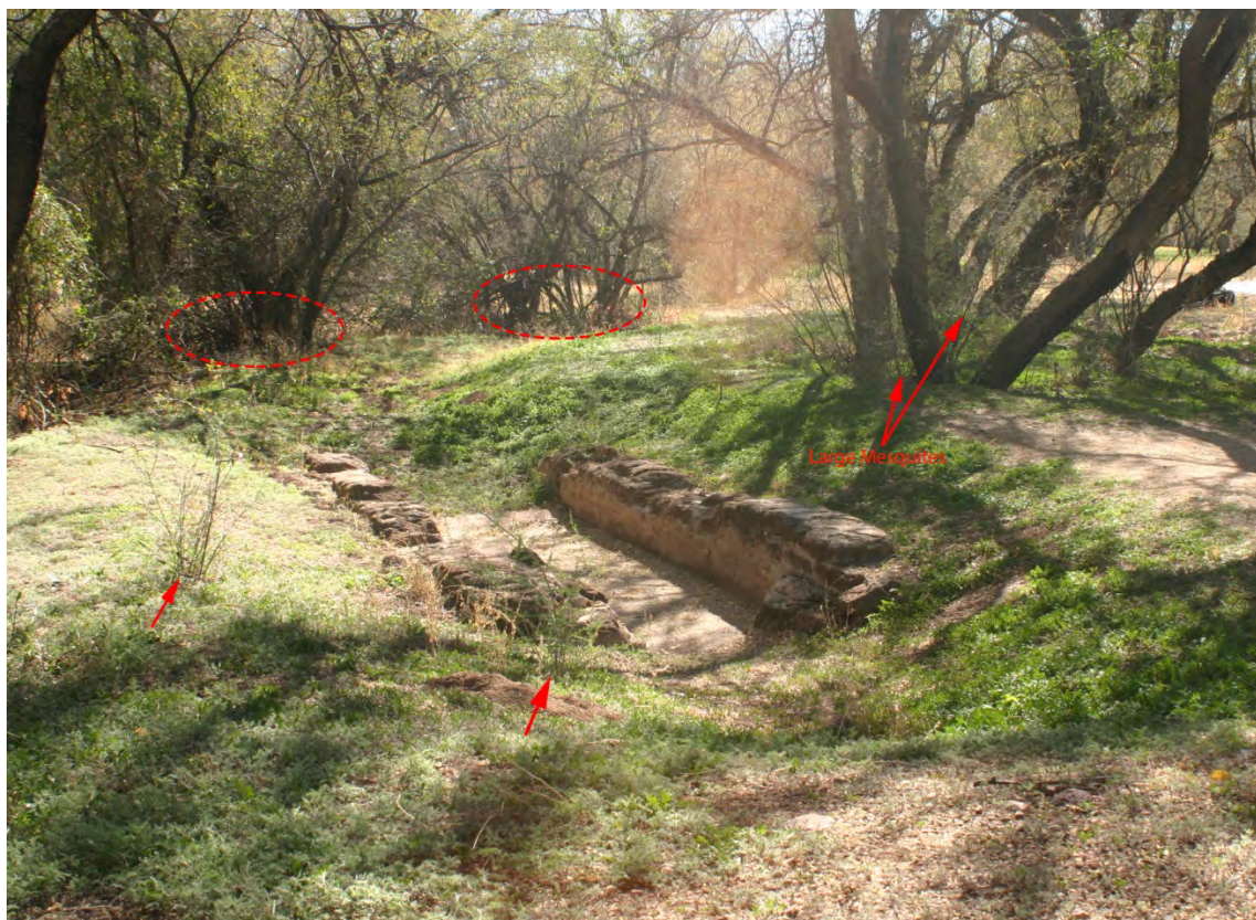
Figure 3.3. Overview of vegetation encroachment: areas of heavy vegetation circled in dashed line; looking south (photographed January 29, 2014).
