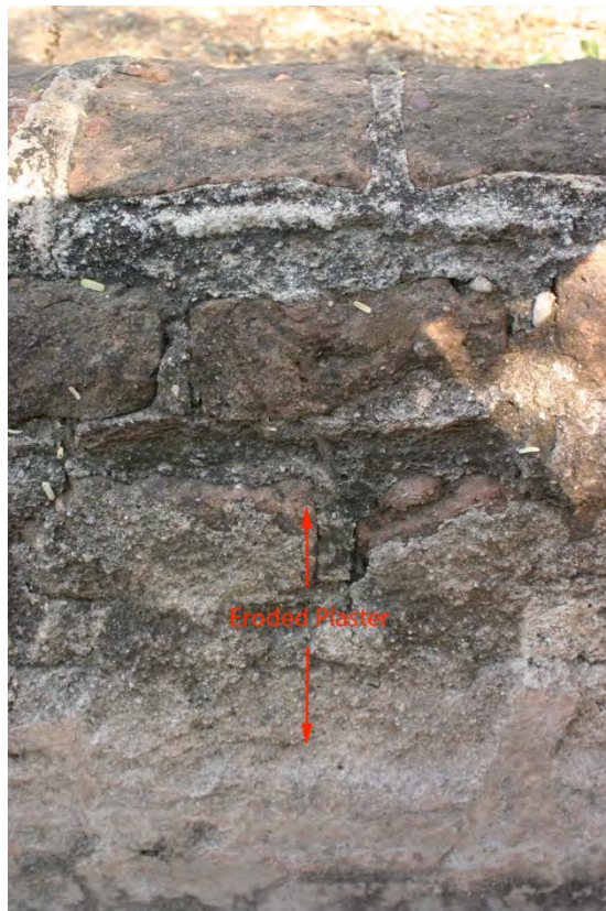
Figure 3.19. Plaster finish on the interior surface of the compuerta has spalled and eroded (photographed November 19, 2013).
