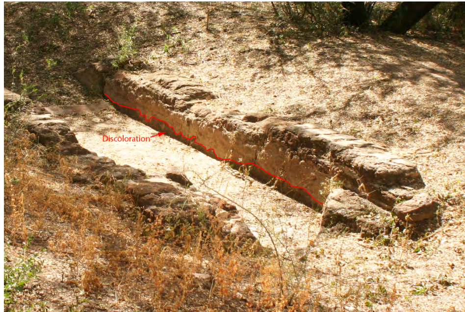
Figure 3.25. Overview of discoloration at base of west wall highlighted in red (photograph looking south, November 19, 2013)
