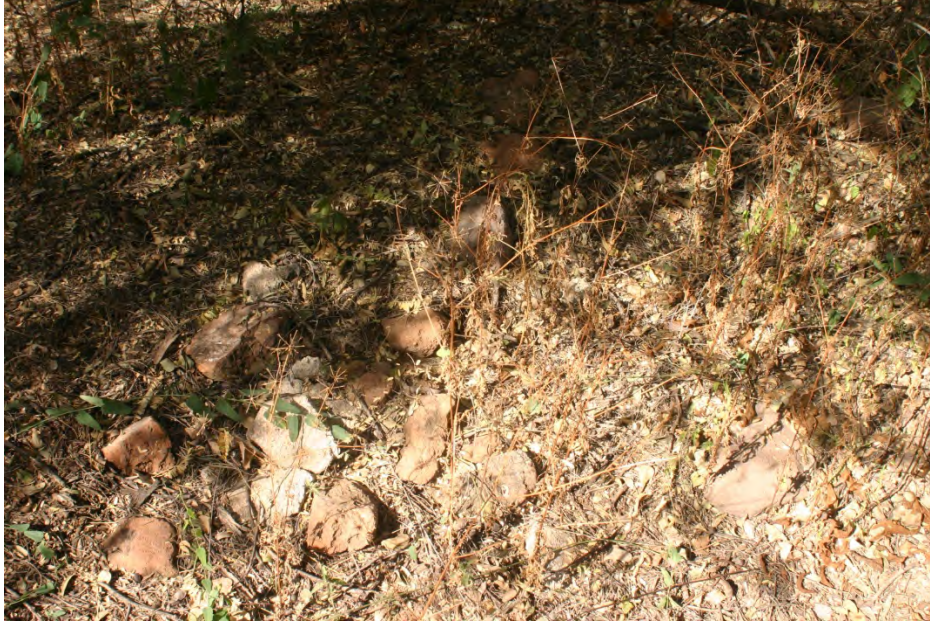
Figure 3.22. Brick and bedding mortar fragments piled to the southeast of the compuerta (photograph facing east, November 19, 2013).
