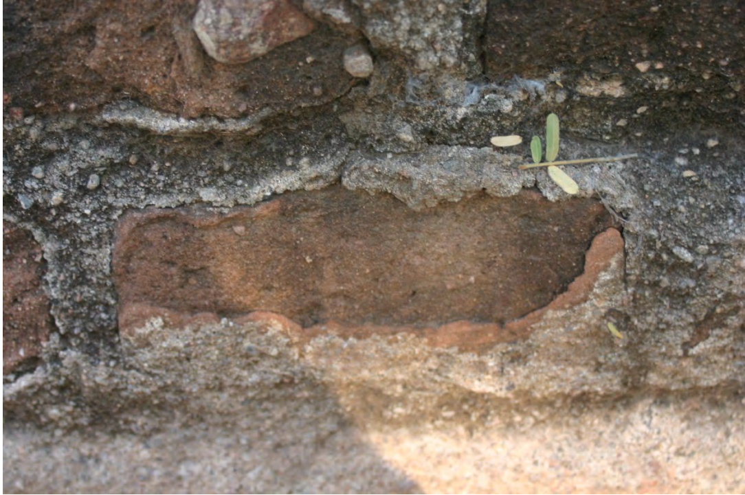
Figure 3.16. Detail of spalled surface on brick, east wall of compuerta (photographed November 19, 2013).
