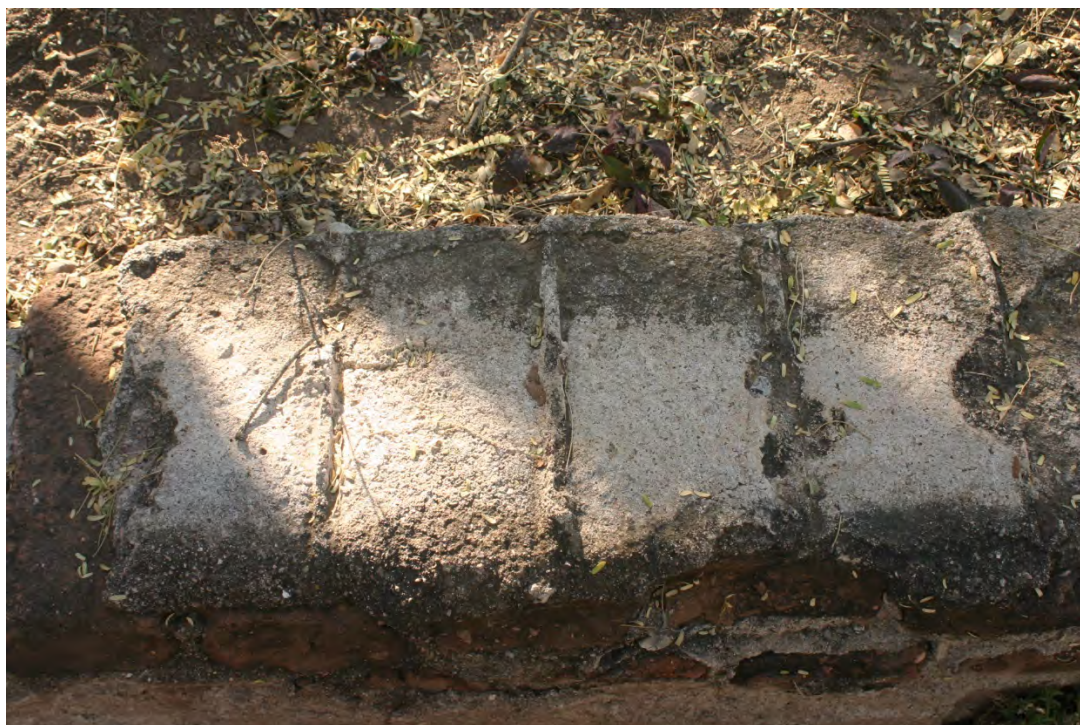
Figure 3.15. Evidence of lost course of bricks at top of compuerta walls, indicated by brick impressions in bedding mortar (photographed November 19, 2014).
