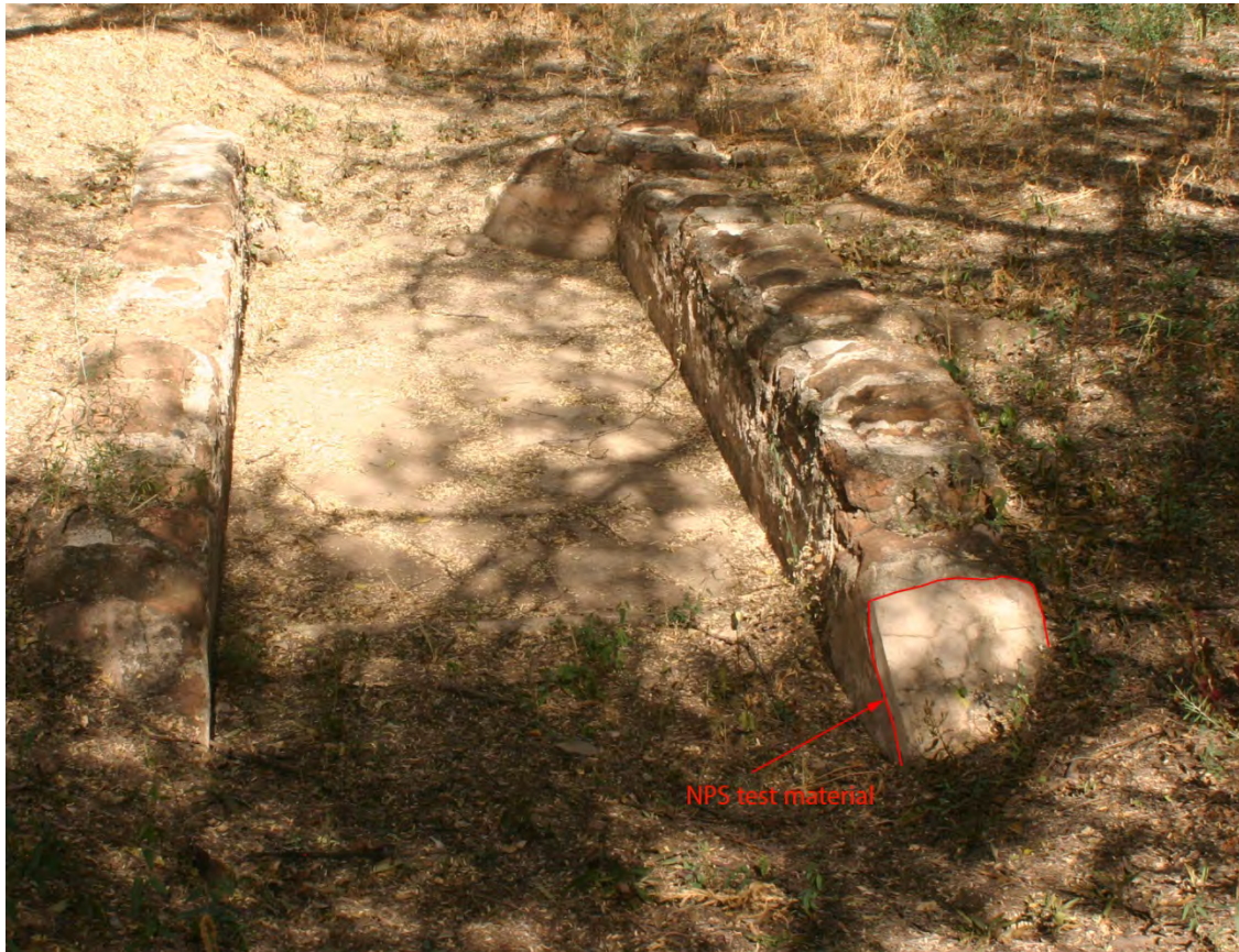
Figure 3.27. Natural hydraulic lime plaster test material at southern end of east compuerta wall (photograph looking north November 19, 2013)
