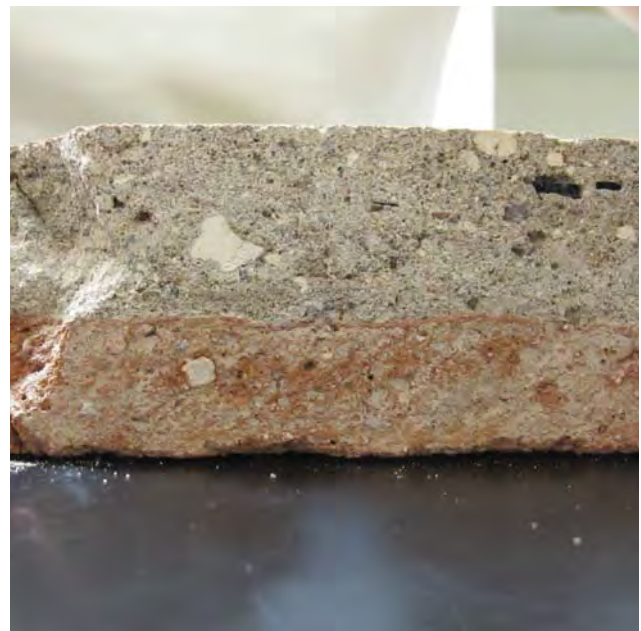
Figure 22: Original plaster with embedded brick surface finish (bottom)
