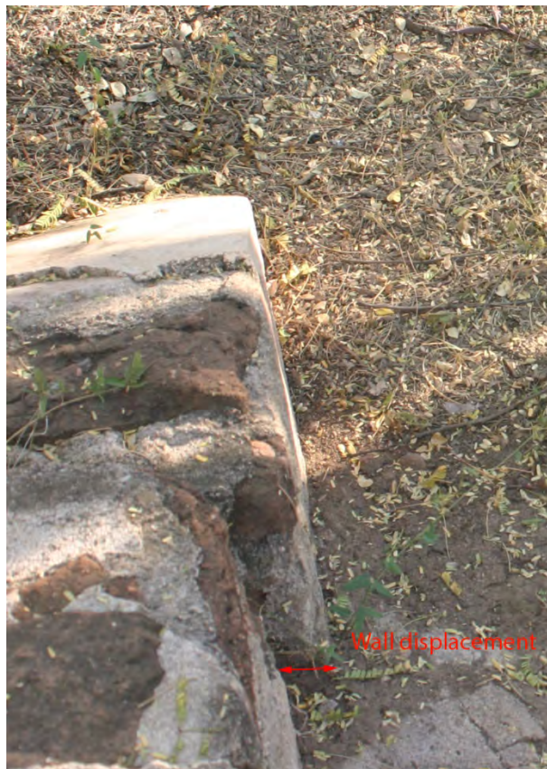
Figure 3.14. Detail of southern end of east wall with displacement of section of wall toward the west (photographed November 19, 2013).
