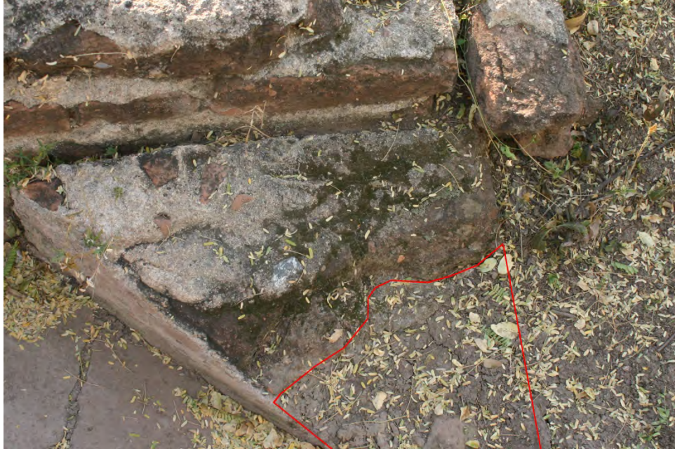
Figure 3.18. Material loss on western portion of weir at northern end of compuerta. Estimated extant of original material lost outlined in red (photographed facing west, November 19, 2013).
