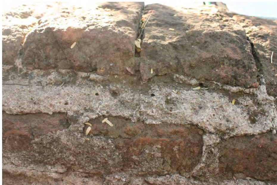
Figure 3.26. Detail of bio-organic growth on the surface of brick and bedding mortar of west wall (photograph November 19, 2013).
