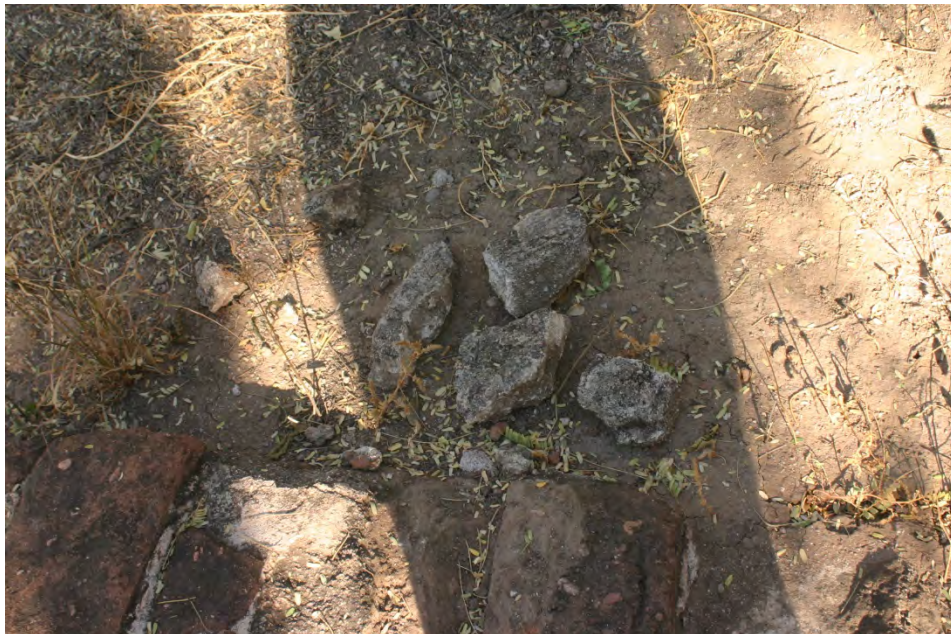
Figure 3.21. Bedding mortar fragments piled near the eastern wall of the compuerta (photograph facing east, November 19, 2013).
