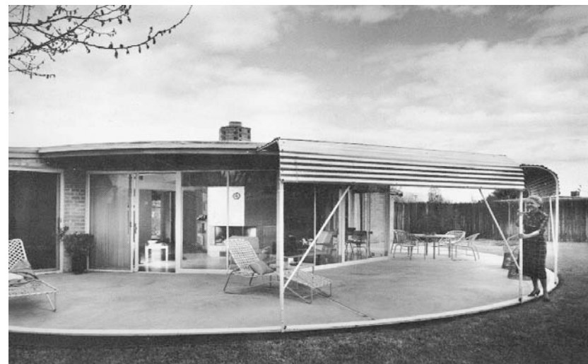
The Ball/Paylore house featured movable corrugated-aluminum shade screens on a track around the patio.
