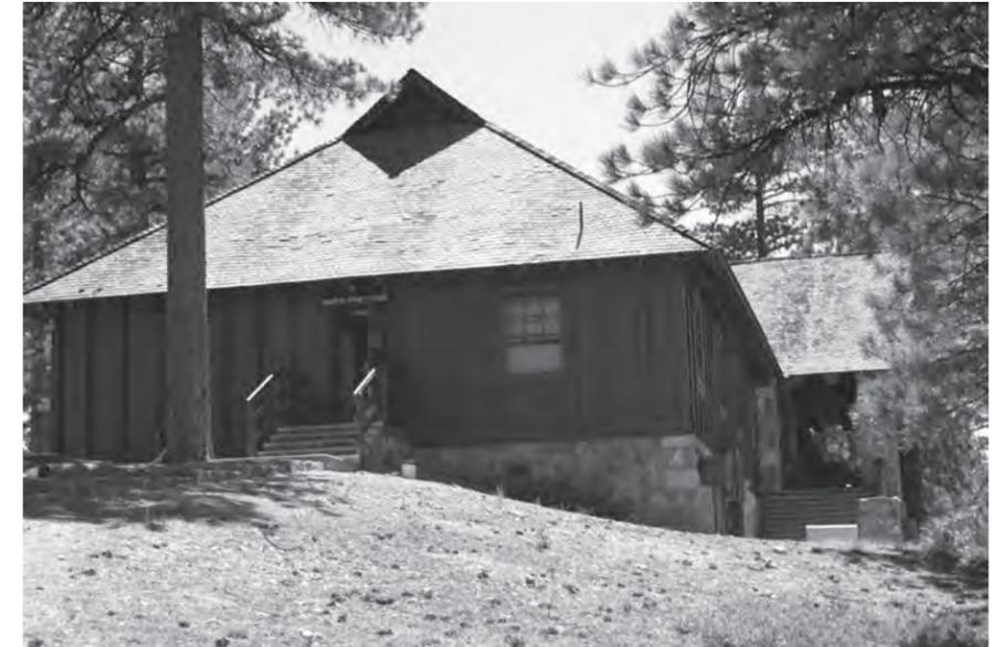
Photograph R/16. The current entry bypasses the main building entrance (to the right in the photo) and uses the side entrance as primary building access. The original entrance should be reclaimed through the installation of a new pathway.
