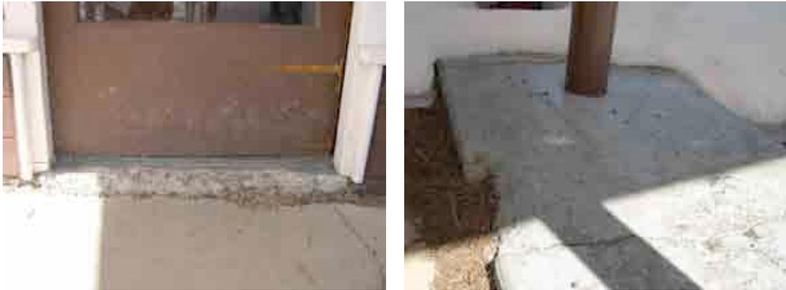
Figure 15 & Figure 16 - Areas of concrete slab cracking and minor loss around the building exterior.
