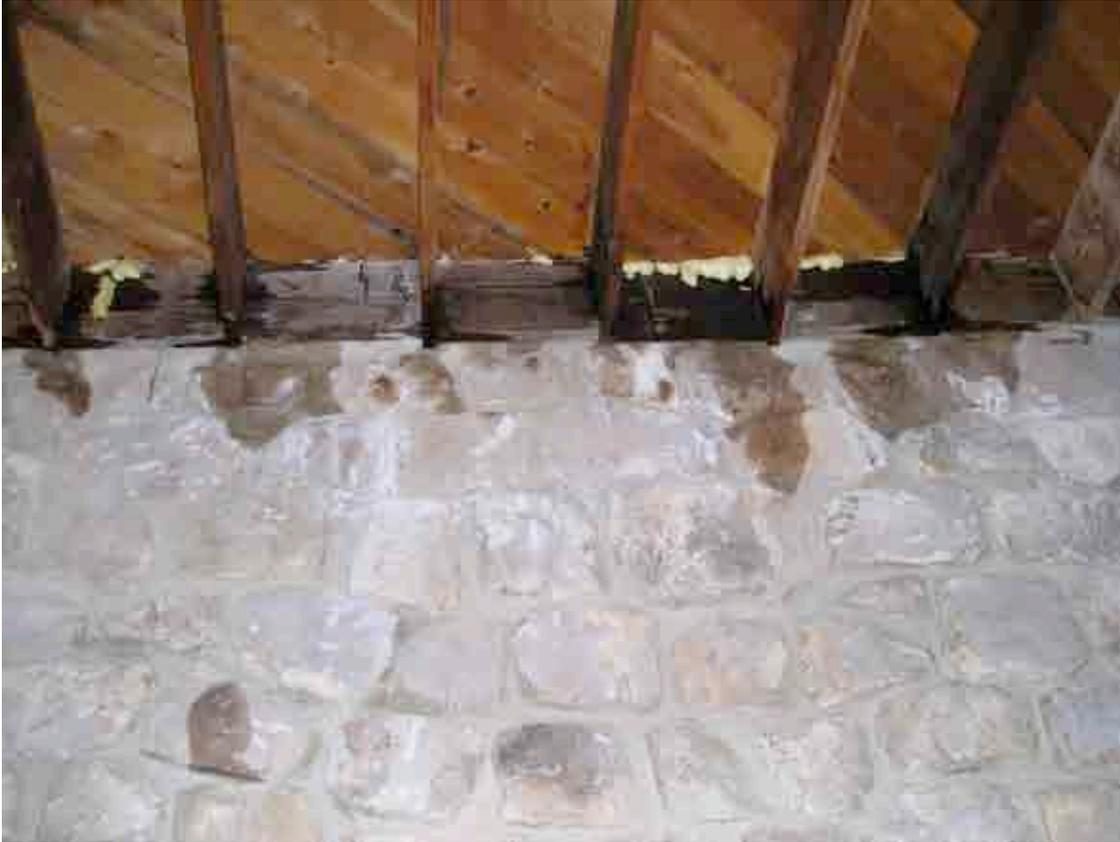
Figure 13 - Water leakage in the interior of the Utility Room between the stone wall and roof plane caused by poor water drainage and inappropriate flashing at connection between stone wall and built-up roofing membrane.
