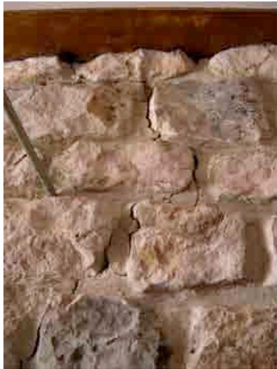
Figure 17 & Figure 18 - Large crack in rear stone wall, exterior (left) and interior (right, in Women's Restroom).
