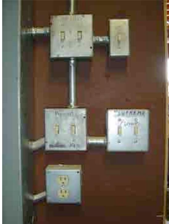
Figure 30 & Figure 31 – Original electrical outlet in Repair Shop using conduit embedded in concrete slab (left) and non-functioning switch boxes in Utility Room (right).
