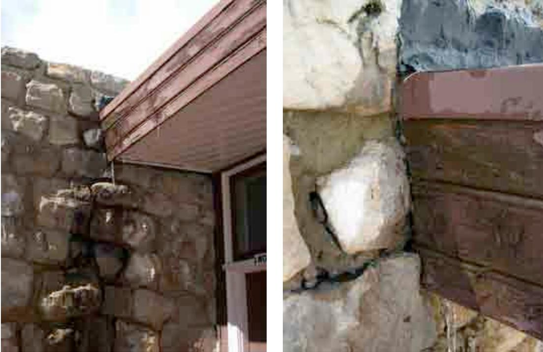
*Figure 7 & Figure 8 - Poor drainage at the southwest corner of the building showing water damage to the stone wall and the fascia.*
