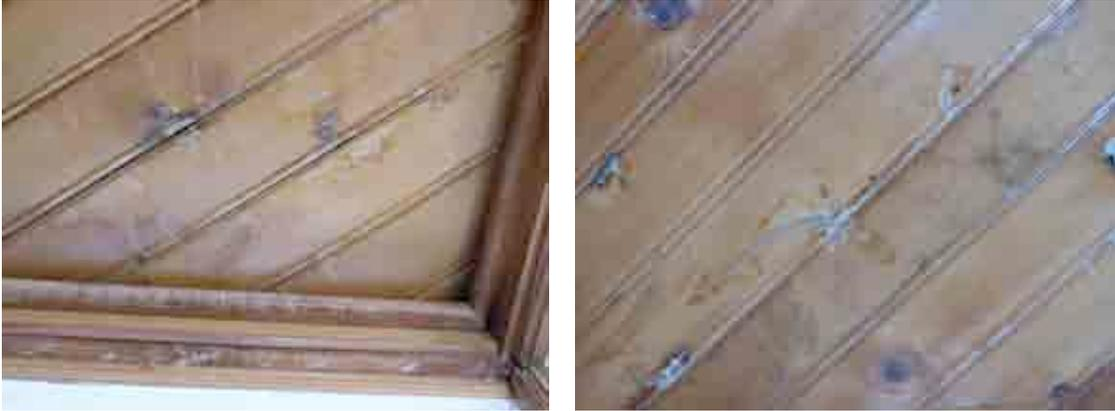
Figure 62 & Figure 63 - Water damage to paneled ceiling and wood trim.
