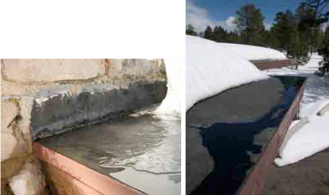
*Figure 5 & Figure 6 - Water ponding on the roof causing damage to the stone wall and at the roof's edge adjacent to the fascia.*
