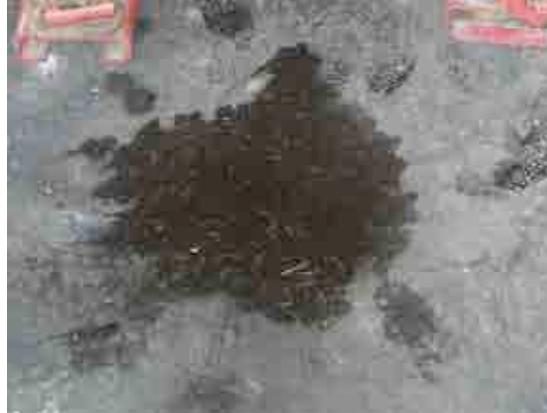
Figure 70 & Figure 71 - Abandoned pulley from garage door mechanism attached to roof joist (left) and fresh oil stains on concrete slab floor from automobile lift.
