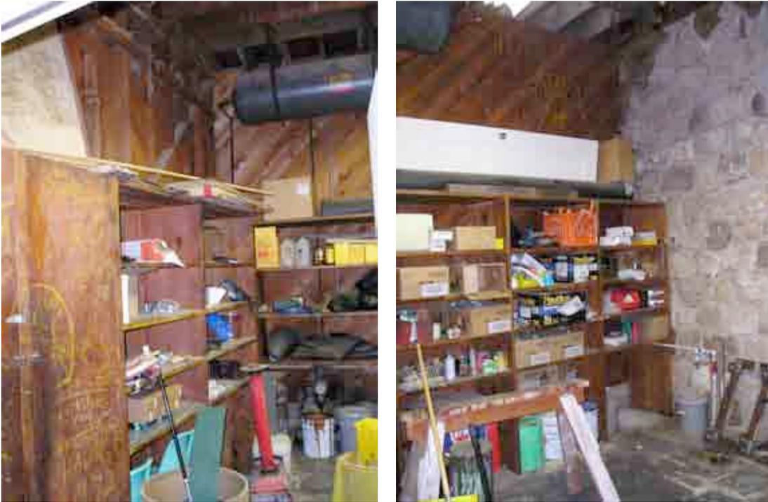
*Figure 73 & Figure 74 - Cabinets on east and south walls showing the compressed air tank, exposed framing of the east wall, diagonal wood paneling of the south wall and the water stains at the connection between the stone wall and roof joists.*
