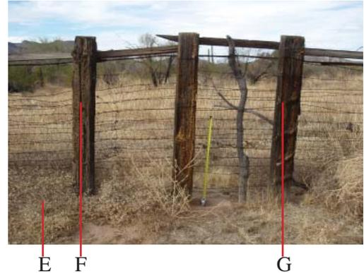
4: Densely spaced vertical mesquite posts & railroad ties with barbed wire & metal piping
