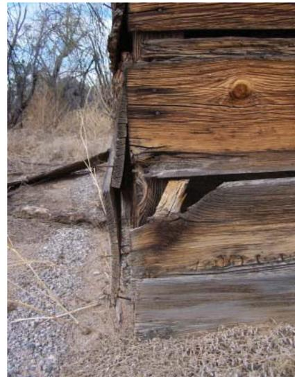
*A,B,C. Water damage to wood paneling and fascia including warping and splintering & rotting due to microorganisms/ pests.*
