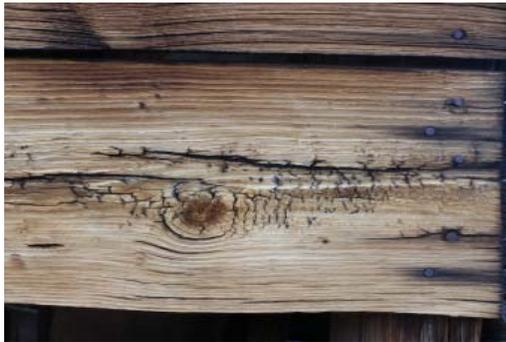
*B. Rotting of wood due to microorganisms/ pests (also termite) infestation.*
