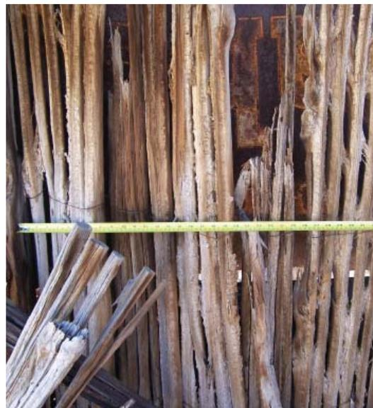
*View of the saguaro ribs tied with barbed wire that make up the walls of the shed.*
