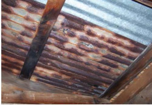
*E. Rusting of the corrugated metal roof due to water damage*
