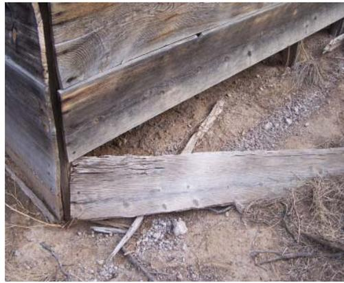
*J. Falling apart of the wooden planks near the base of the structure.*
