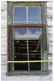
*M. View of the window on north wall. Note the new frame nailed on top .*
