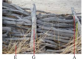
3: Regularly spaced vertical mesquite posts with barbed wire & metal piping
