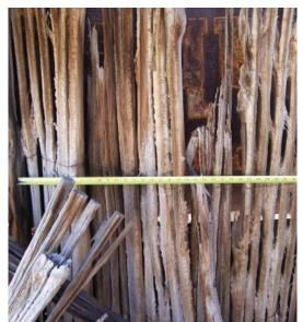
View of the saguaro ribs tied with barbed wire that make up the walls of the shed.
