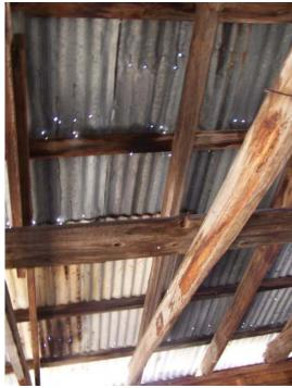
*E.* Detail view of metal roofing from the interior. Notice the rusting of sheets.
