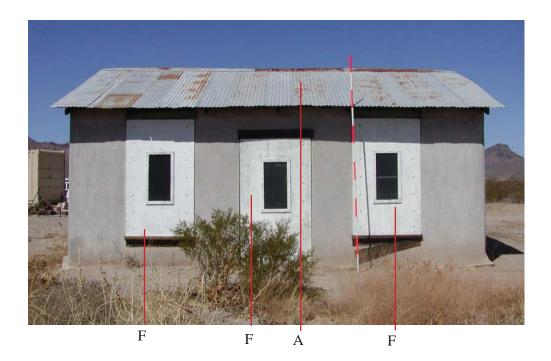
*Fig. 3 - South elevation of the Main Residence (letters refer to notes in condition assessment table below)*
