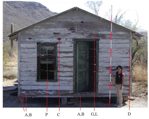
*Fig. 3 - East elevation of the Bunkhouse* (*Letters refer to notes in condition assessment table ahead*)
