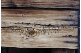
*B.* Rotting of wood due to microorganisms/ pests (also termite) infestation.
