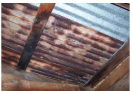
*E. Rusting of the corrugated metal roof due to water damage*
