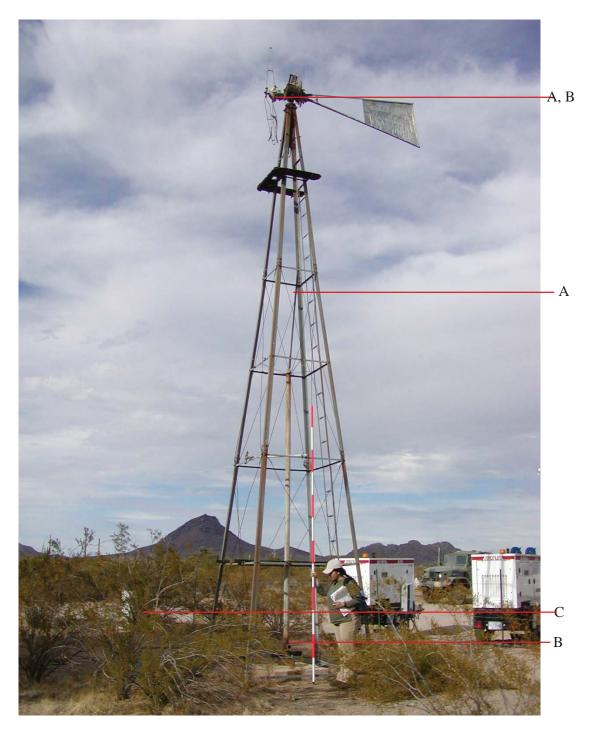
Fig 1. View of Windmill #1 from the south side showing existing damages and deficiencies. (letters refer to notes in condition assessment table below)
