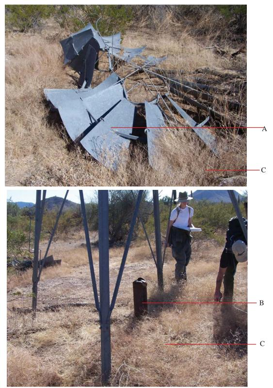
*Fig. 4 - Blades from Windmill#3 lie on the ground near its base. (letters indicate damages and deficiencies based on table that follows*
