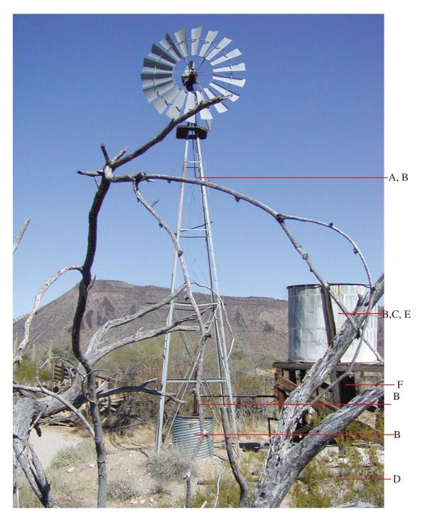
*Fig 3. View of Windmill #2 from the west side showing existing damages and deficiencies. (letters refer to notes in condition assessment table below)*
