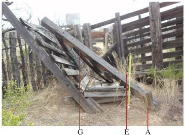
Fig. 5 - East elevation of the shade structure (letters refer to notes in condition assessment table)
