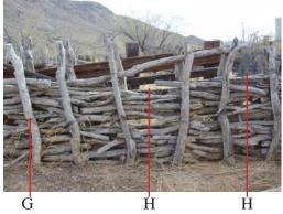
2: Horizontally stacked mesquite logs & regularly spaced vertical mesquite posts, collapsed
