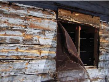
*M*, *A*, *B*. Detail view of window on west elevation. Note the wire mesh screen coming off & new board above
