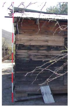
J. Detail view of north facade. Note the plank that is falling apart off near the base of the structure
