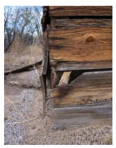
A,B,C. Water damage to wood paneling and facia including warping and splintering & rotting due to microorganisms/ pests.
