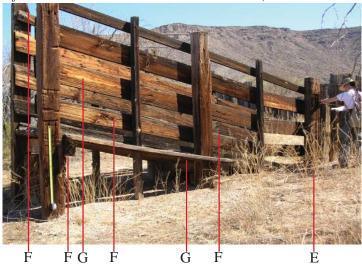
*Fig. 4 - Southeast elevation of the shade structure (letters refer to notes in condition assessment table)*
