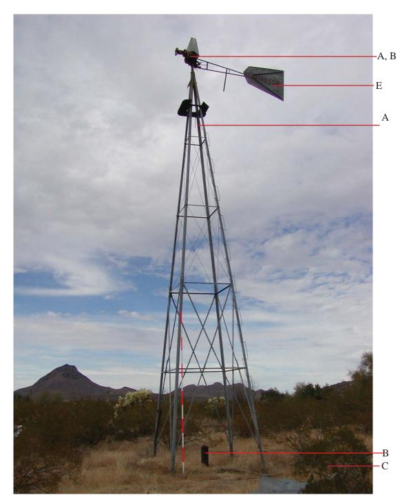
*Fig 3. View of Windmill #3 from the south-west side showing existing damages and deficiencies. (letters refer to notes in condition assessment table below)*
