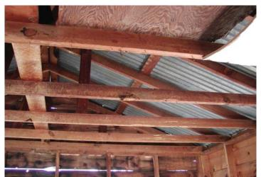
*View of the roof trusses. Note the relatively new metal sheeting on the roof*
