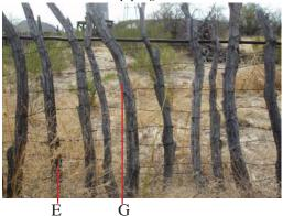
4: Densly spaced vertical mesquite posts & railroad ties with barbed wire & metal piping
