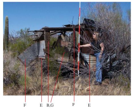
*Fig. East elevation of the Ocotillo Shed* (*Letters refer to notes in condition assessment table ahead*)
