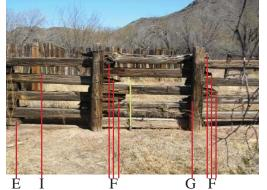
3: Horizontally stacked mesquite logs with irregularly spaced vertical mesquite supports
