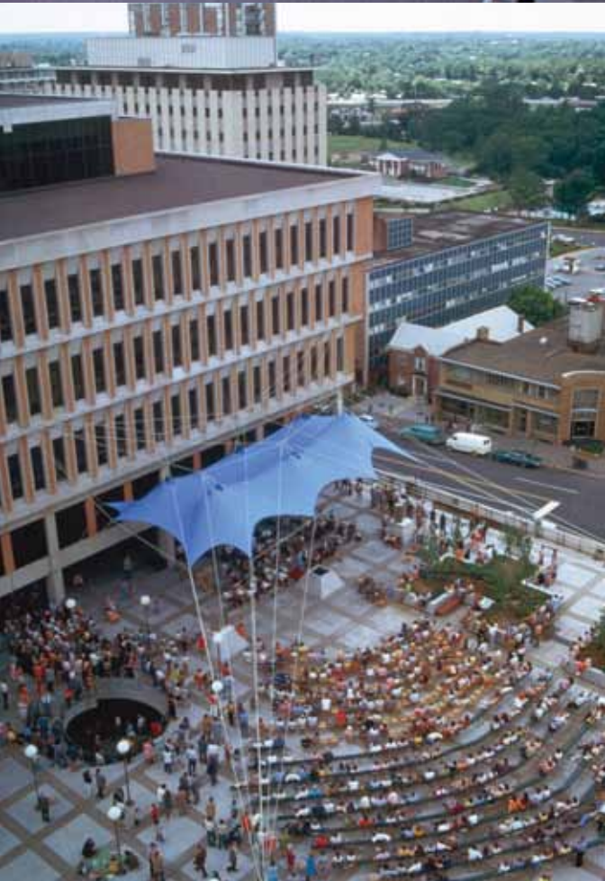
图 5. Stretch fabric temporarily suspended from adjacent buildings shades St. Louis Symphony during mid-day concert.
