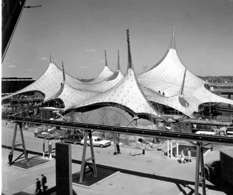
图 1. German Pavilion at Expo 67 Montreal, fabric membrane suspended below steel cable network.
