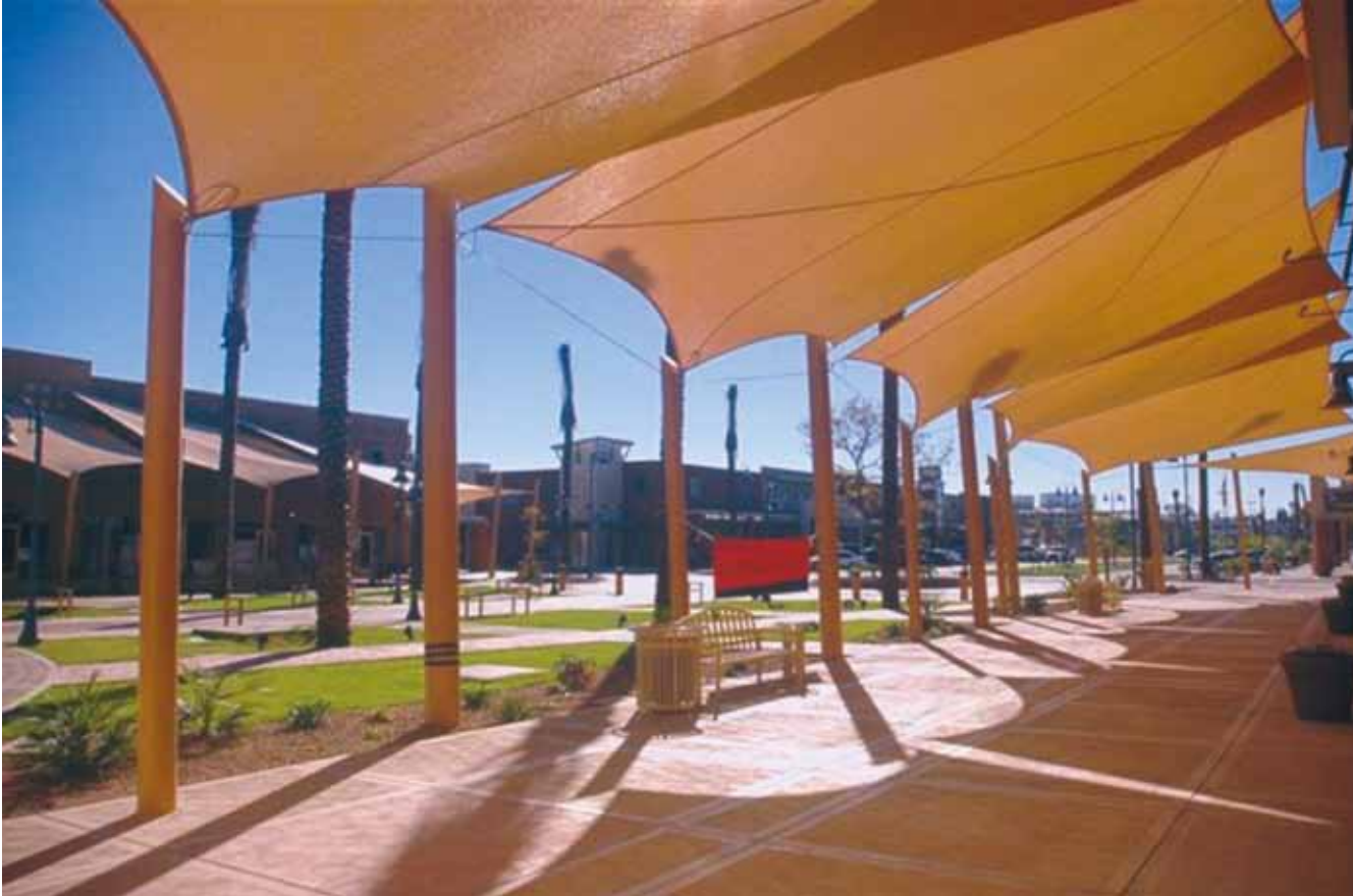
图 9. At the Yuma Palms Shopping Center HDPE mesh fabric canopies along both sides of the outdoor mall insure that a shaded walkway is always available. Yuma Palms 购物中心, 高密度聚乙烯网状织物膜铺设两边街道商店外面的人行道上, 保证行人在阴影中通行。
