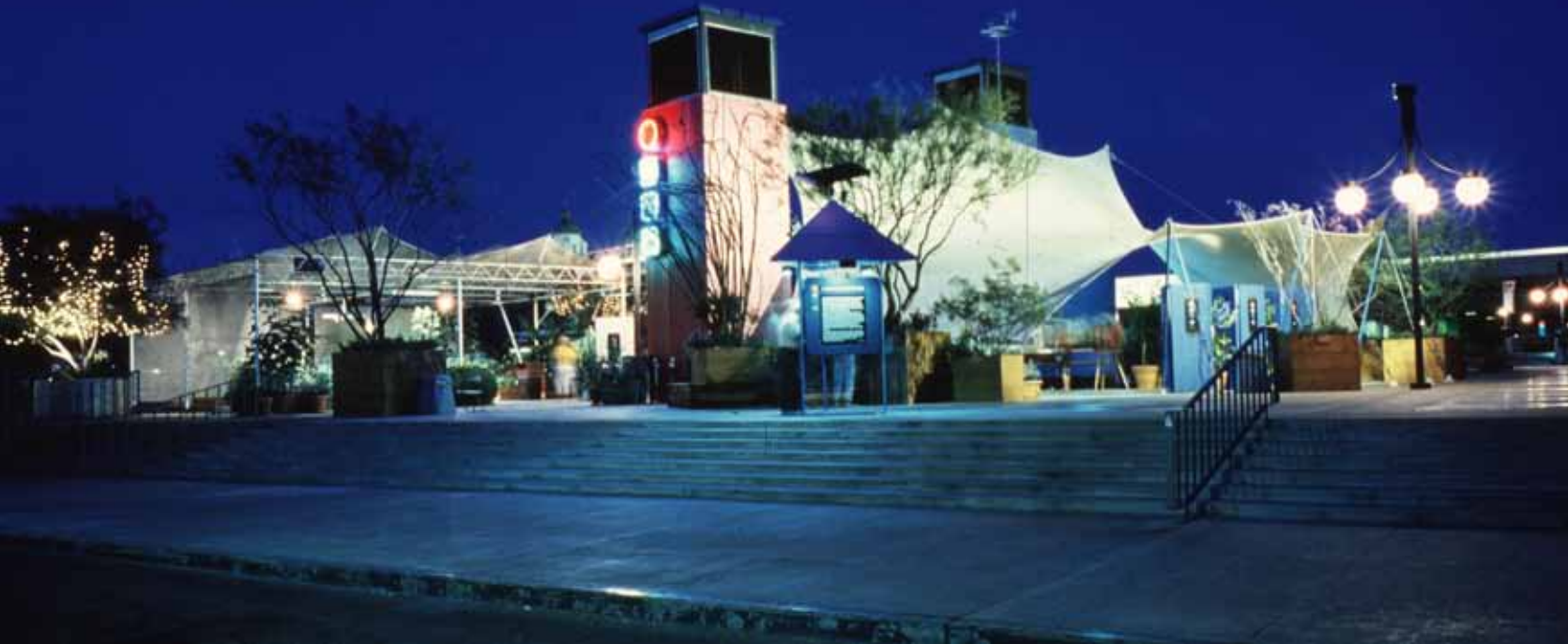
图 11. At the “Summer Invitation” Phoenix Civic Plaza, the tensile membrane is shaped to create cool breezes under the canopy.
