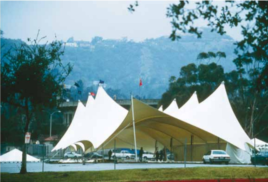
图 17. A modular pavilion can be set up with two or more modules to accommodate small to very large events.
