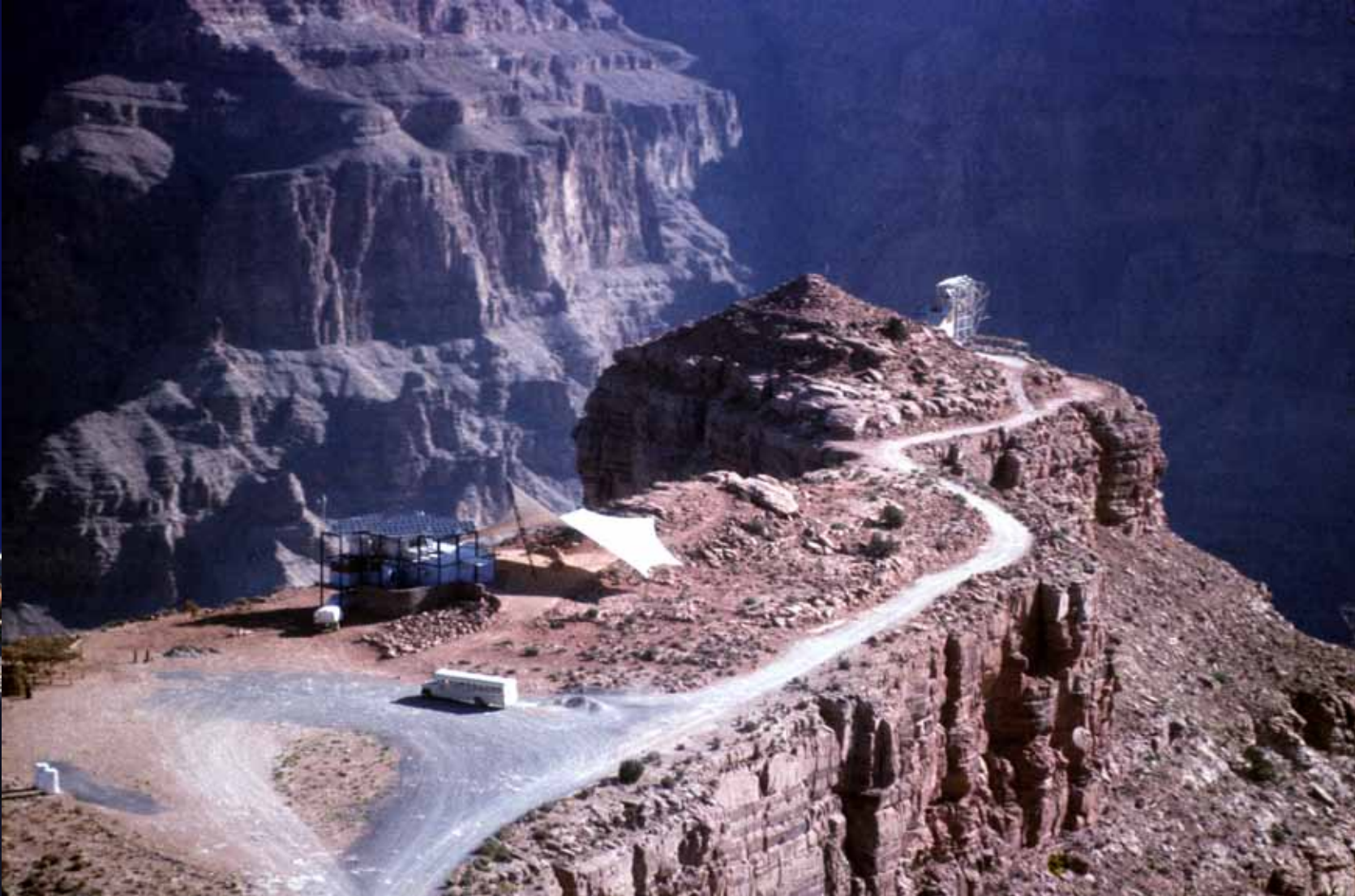
图 12. At the Hualapai Nation Grand Canyon West Visitor facility, the fabric membrane is shaped to shade summer sun, but admit lower winter sun.
