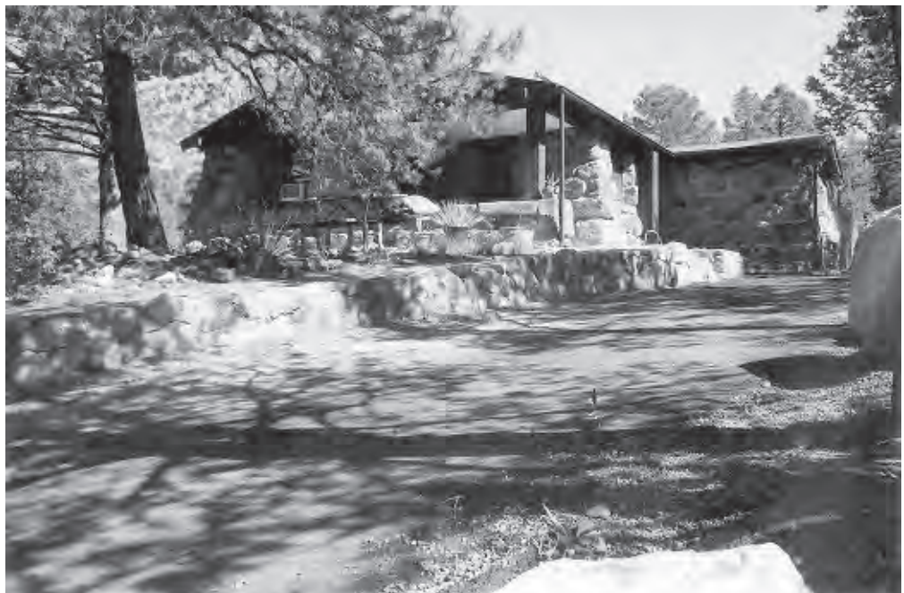
Figure 136. Recent image of Residence #3 illustrates changes to front yard including lowering of driveway and construction of retaining Wall, 2002. View looking east.
