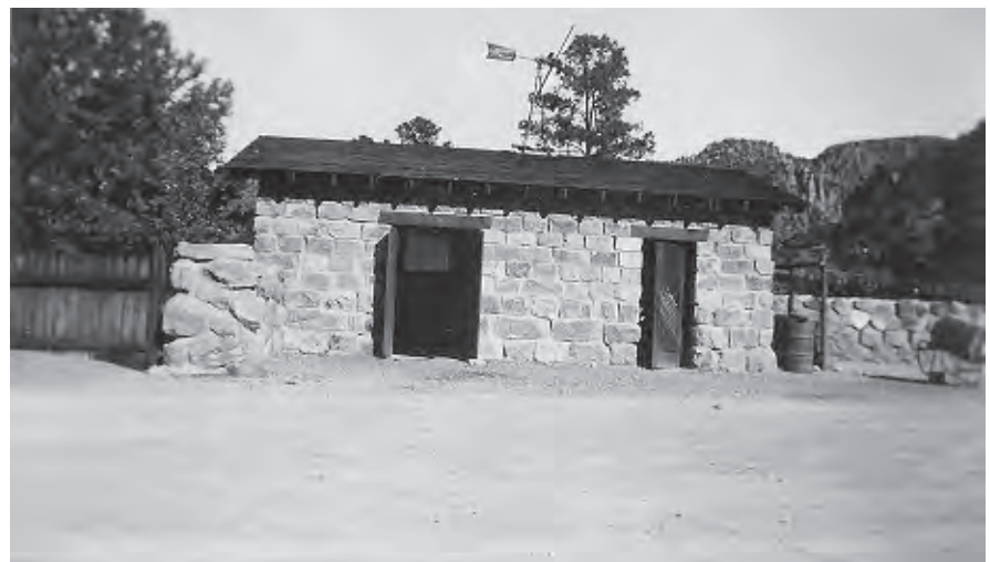
Figure 126. The south face of the Power House and Laundry walls are composed of rectangular cut block and show little batter, 1949. Note the wooden stockade on the left hand side. View looking north.
