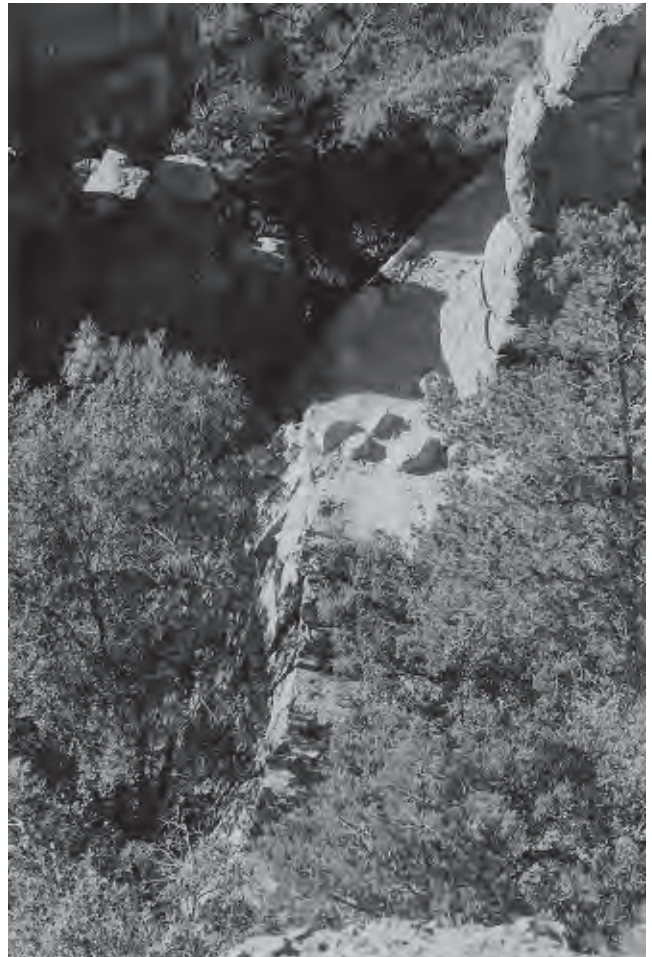
Figure 31. Large retaining walls on upper Sarah Deming trail, 2003.
