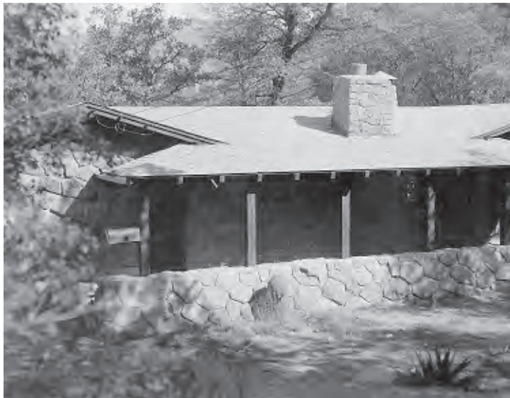
Figure 76. Rear porch and entry to Administration Building, 1960. View looking northeast.
