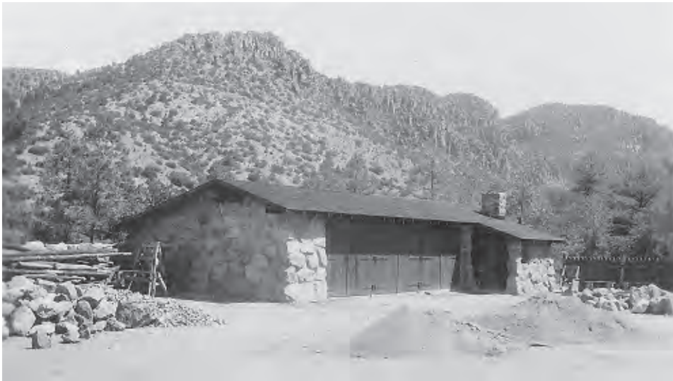
Figure 123. Warehouse shortly after construction with three bays and 'ell' at south-east corner, 1939. Note wooden stockade at far right. View looking northeast.
