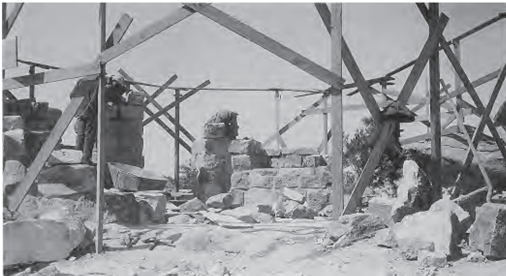
Figure 69. Construction of Orientation Station walls. Note large boulder at right incorporated into Northwest wall. View looking West. 1939.
