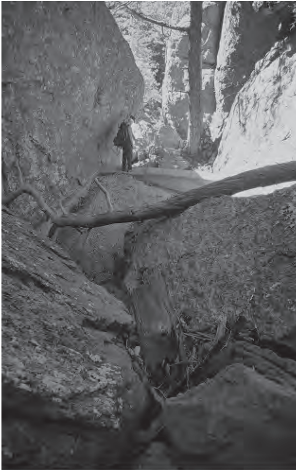
Figure 29. Echo Canyon dam is now filled with sediment, 2004.
