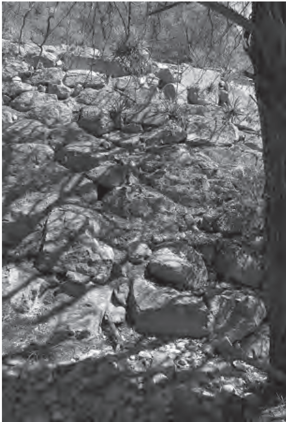
Figure 12. Riprap along Bonita Canyon Creek, 2004.
