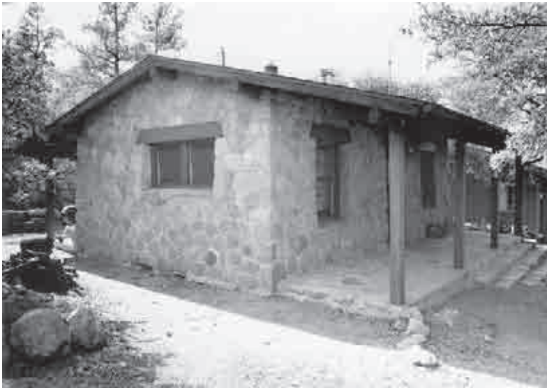
Figure 131. Stone-veneered front porch of Residence #2, 1993. View looking southwest.
