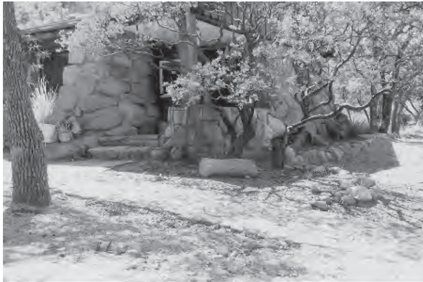
Figure 127. Porch entrance to Ranger Residence #1, 2002. Stonemasonry includes strongly battered walls constructed of large, uncut rubble. View looking south.
