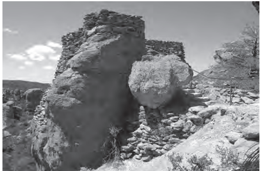
Figure 66. Speakers Rock at Massai Point incorporates large boulders into base of rostrum and boundary of stairs. View looking Northwest. March 2004.
