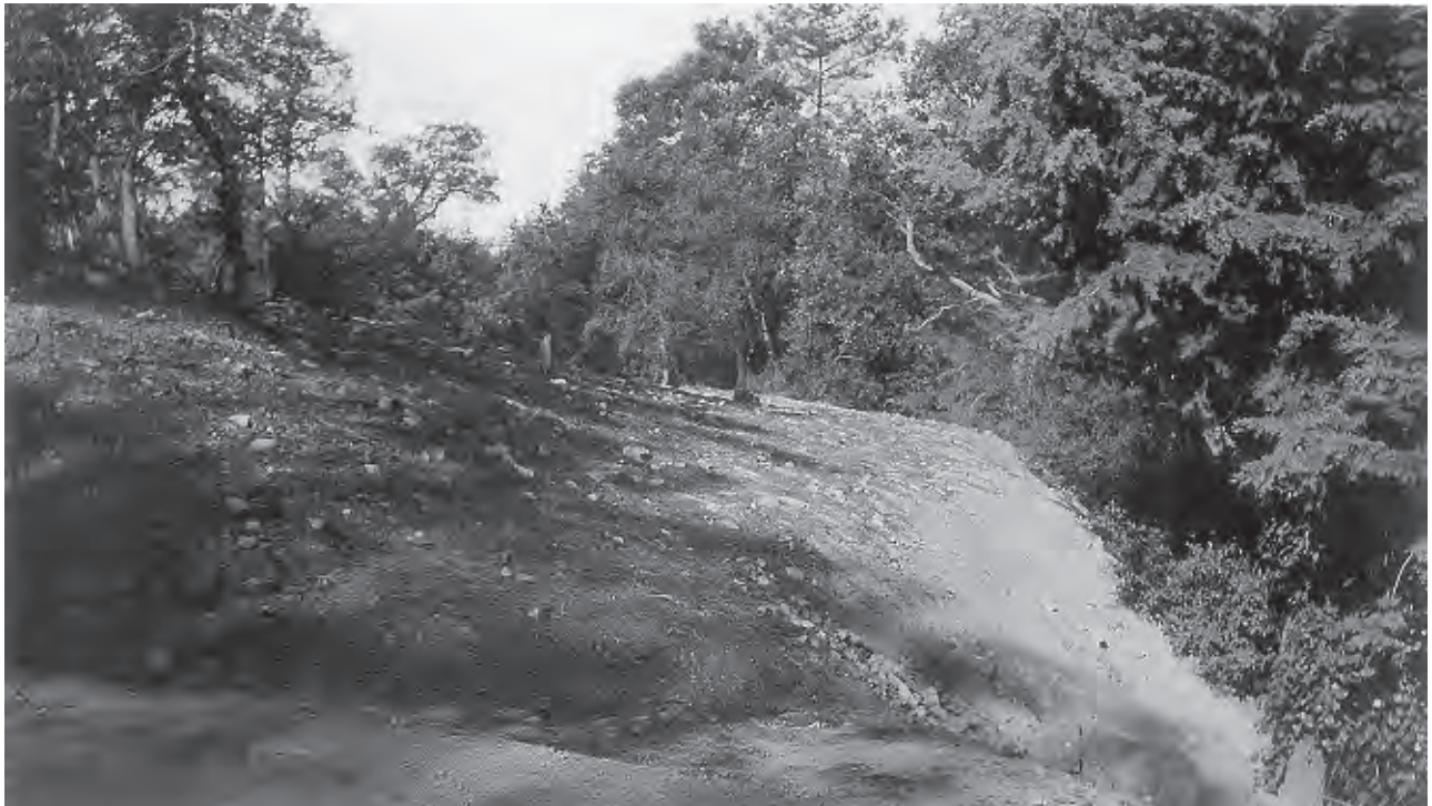
Figure 16. Obliteration of old road completed.
