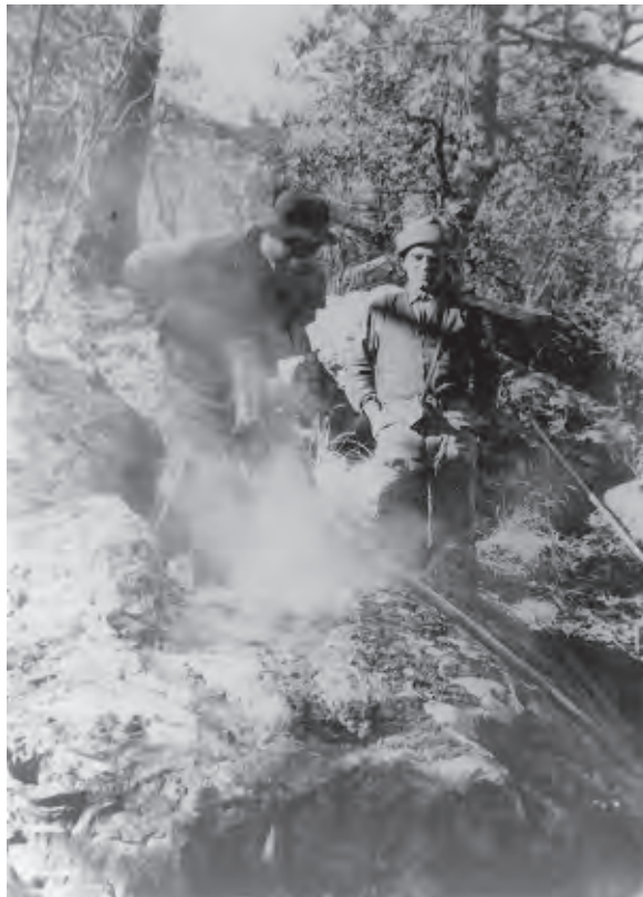
Figure 21. CCC trail crew using air-powered jackhammer to cut through rock.
