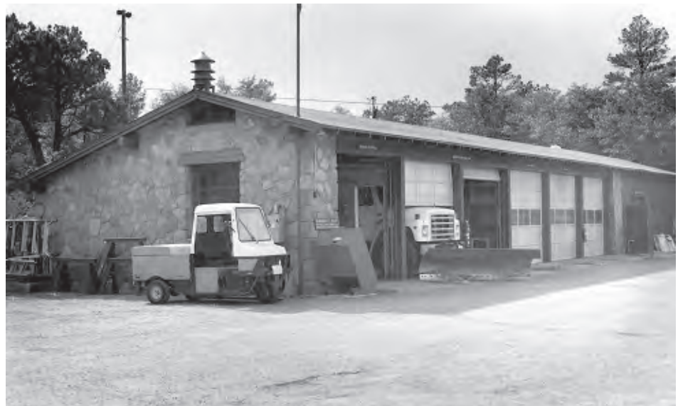
Figure 122. The Equipment Shed with modern pulldown doors and its addition at right, 1993. View looking southwest.
