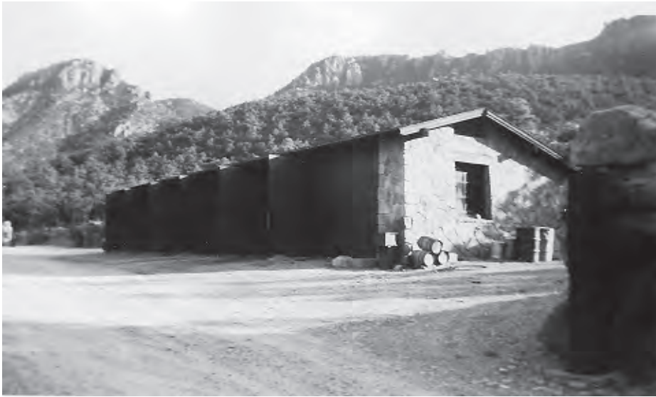
Figure 121. An early image of the Equipment Shed prior to the western addition shows the original bay doors, 1949. View looking southeast.
