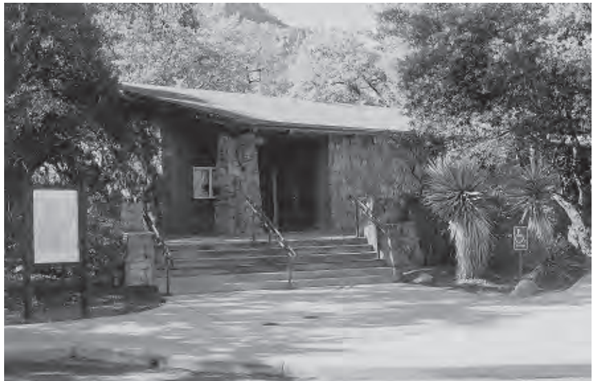
Figure 78. Front entrance to Visitor Center with steps, porch, and stone-veneered walls, 2002. View looking southwest.
