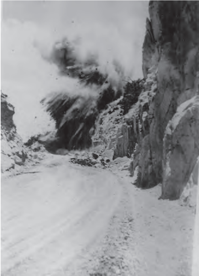
Figure 3. Blasting overhanging rock on Bonita Canyon Highway.
