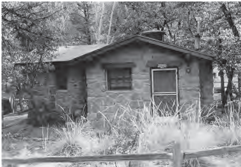
Figure 94. Campground Bath and Laundry House in 1970 was converted to employee residence, 1993. View looking west.
