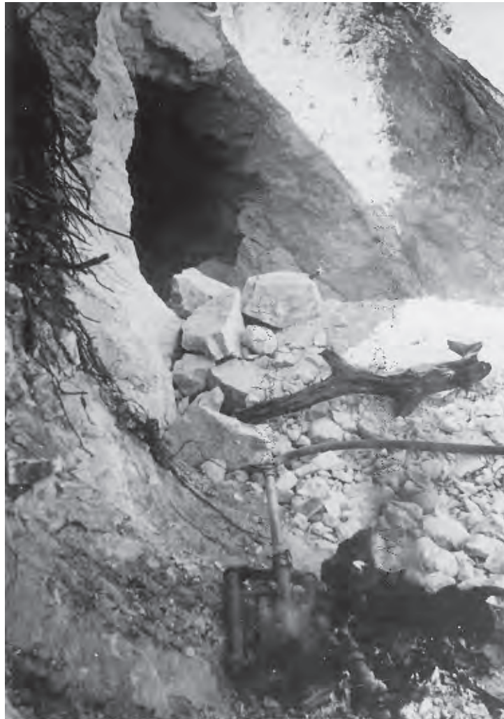
Figure 112. Portable air compressor used for cutting through tunnel on Sugarloaf Trail, 1935.
