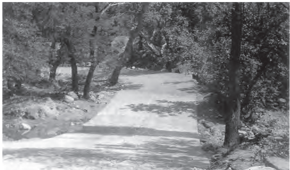
Figure 88. Second concrete dip, 1935. View looking southeast.
