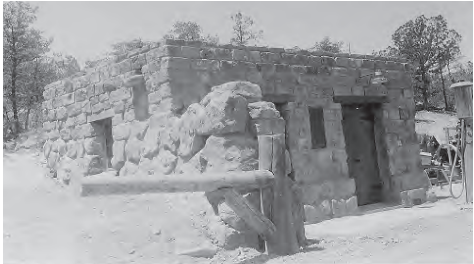
Figure 119. Oil and Gas House, rock pier, and wooden gates at east entrance of the Utility Area, 1939. Note light fixture above door and gas pump on the far right. View looking southwest.
