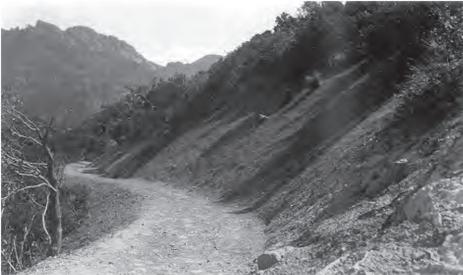
Figure 113. Section of Sugarloaf Trail shortly after completion, 1935. View looking northeast.
