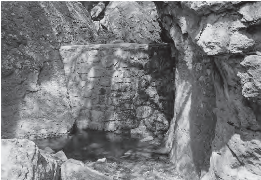
Figure 28. Echo Canyon dam was constructed of concrete and faced with stone, 1993.
