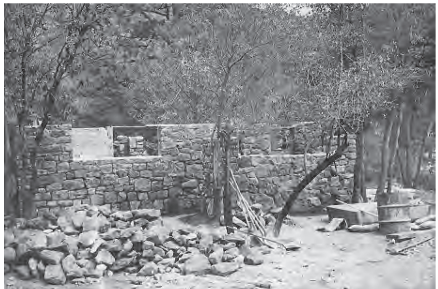
Figure 92. Construction of Campground Comfort Station, 1935. View looking northeast.
