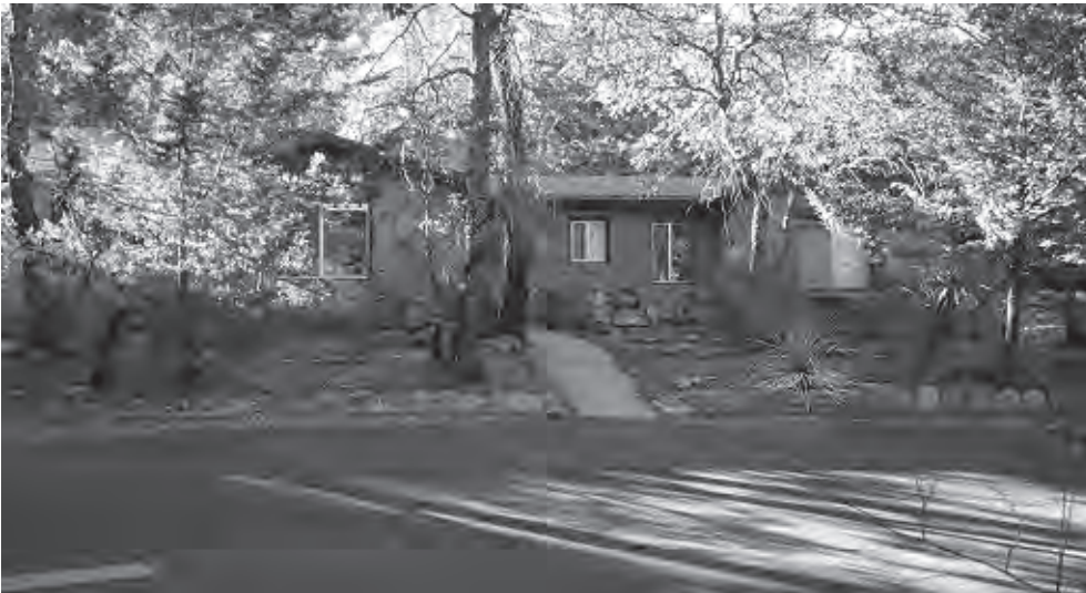
Figure 81. Recent changes to Administration Building include windows, doors, and walkway, 2003. View looking south.
