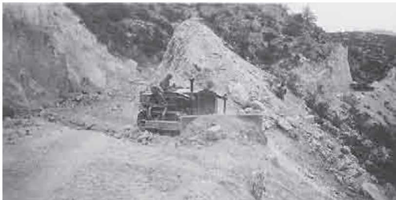
Figure 8. Clearing blasting debris on Bonita Canyon Highway
