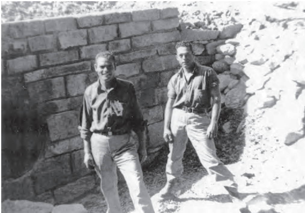
Figure 11. CCC enrollees reconstructed many Bureau of Public Roads culverts.
