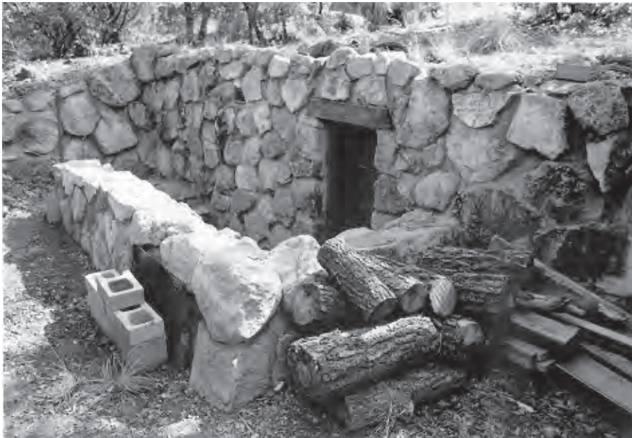
Figure 133. Root cellar in backyard of Residence #2, 1993. View looking south-east.
