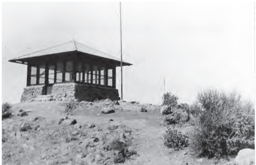
Figure 106. Sugarloaf Lookout illustrates the National Forest Service L-4 design, 1935. View looking southwest.
