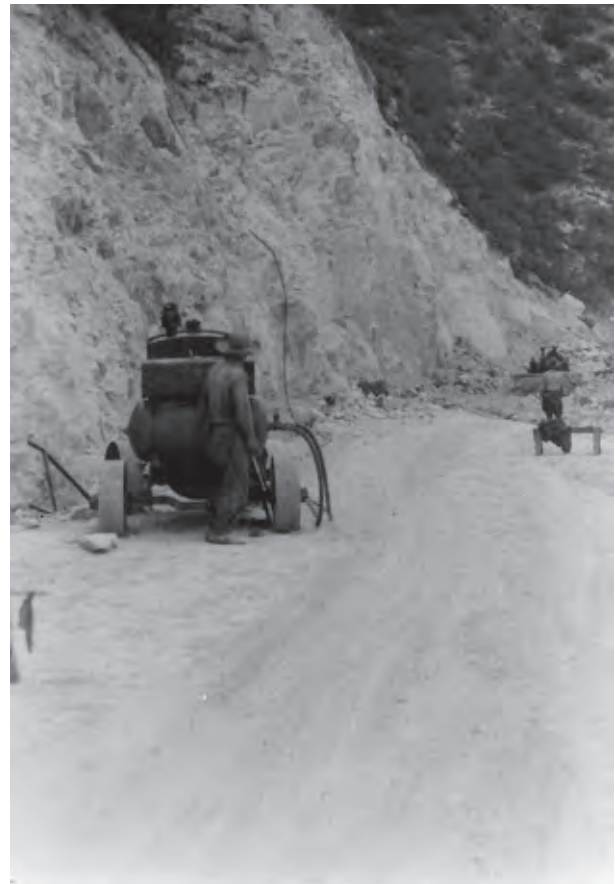
Figure 4. Air compressor used for drilling rock on Bonita Canyon Highway.
