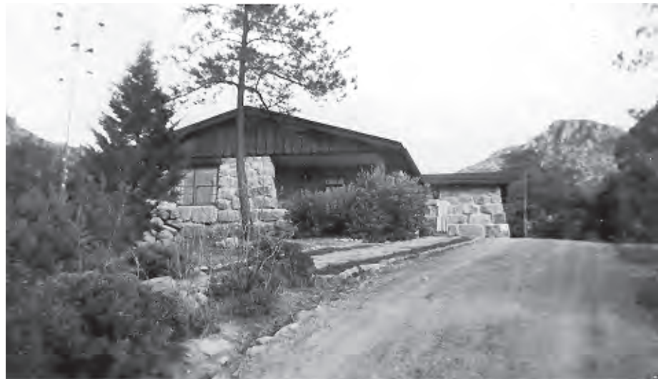
Figure 134. Front of Residence #3 shows stonemasonry with rectangular cut block and strongly battered walls, 1949. Note walkway and vegetation in front yard. View looking east.
