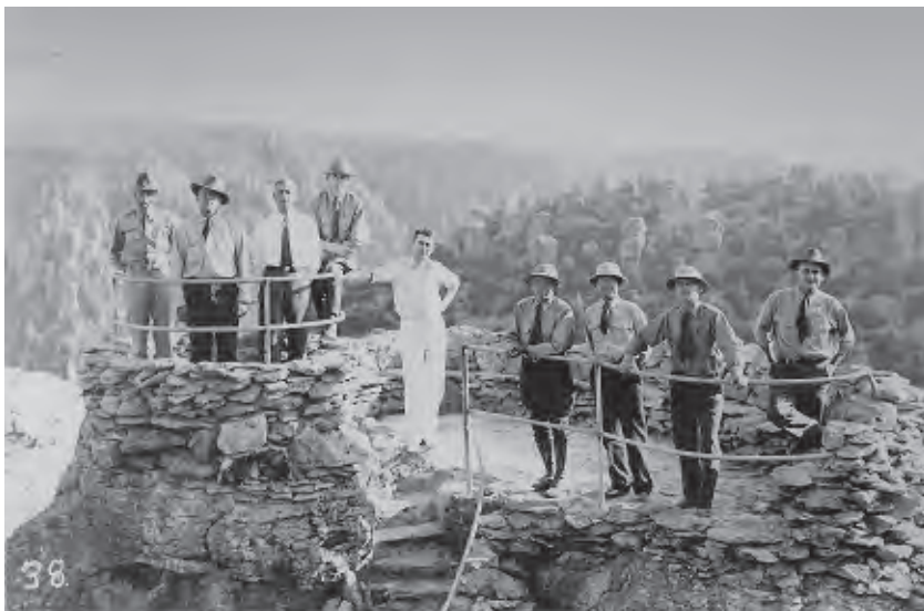
Figure 67. Speakers Rock prior to removal of iron handrails and construction of seating wall on North side. View looking South.
