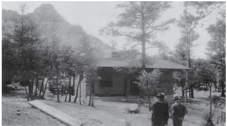
Figure 130. Residence #2, 1939. Note stone retaining wall at left. View looking southwest.
