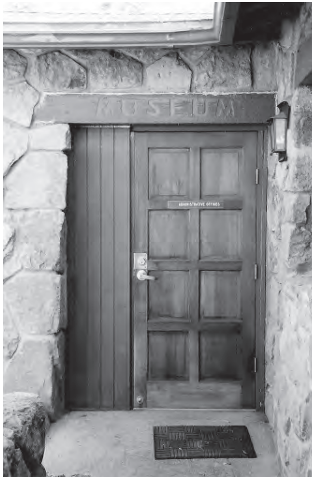
Figure 80. Museum wing double French doors were replaced by a single door after 1965. Note entrance sign carved by CCC carpentry shop in lintel above door, 2002.
