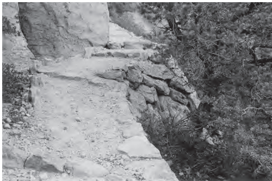
Figure 25. Echo Canyon trail contains numerous constructed features: water bars, retaining walls, and drainage channels, 2002.
