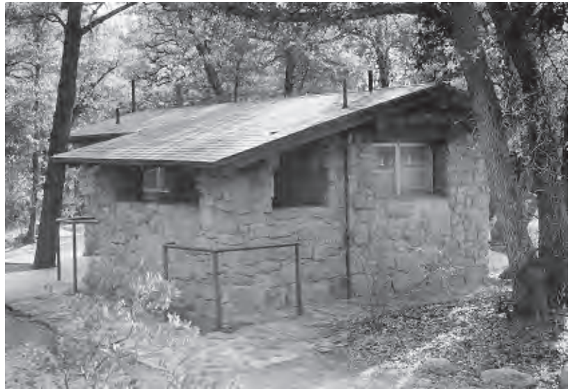
Figure 93. Modern campground comfort station with pathways and handicap access, 1993. View looking southwest.
