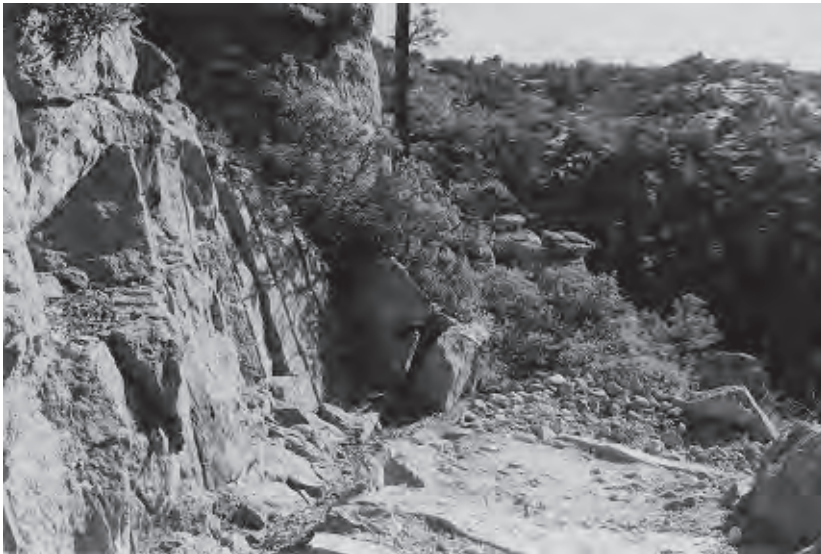
Figure 32. Water bars, drainage channels, and drill marks on upper Sarah Deming trail, 2003.
