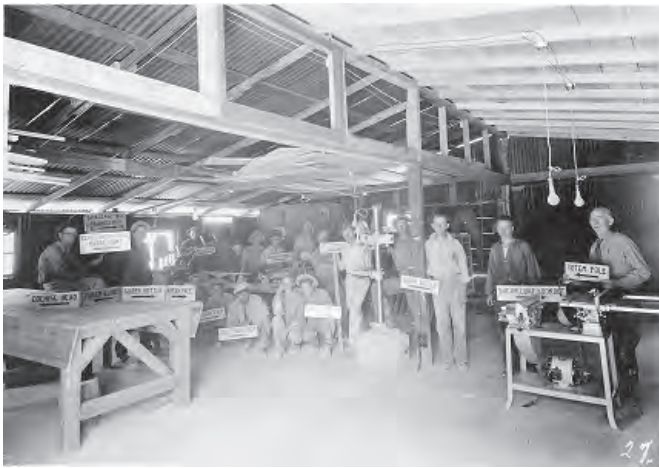
Figure 99. CCC enrollees display trail signage in carpentry shop at CCC Campsite.
