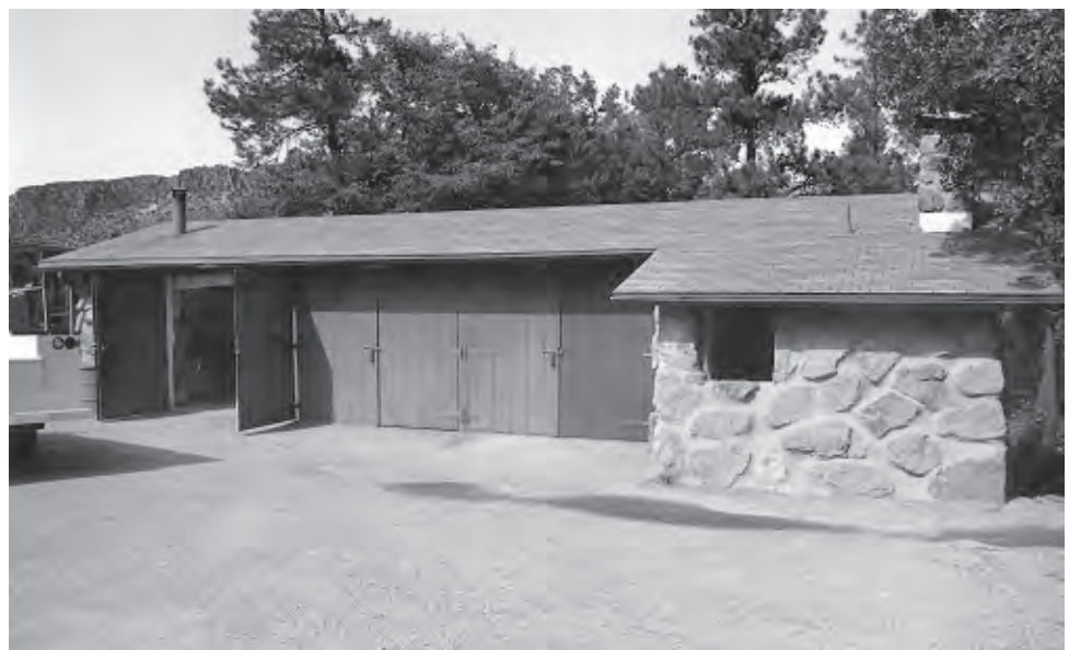
Figure 124. Warehouse with modern bay doors, 1993. Walls are composed of un-coursed stone and are slightly battered. Note the decreasing size of stone from the foundation up. View looking northwest.
