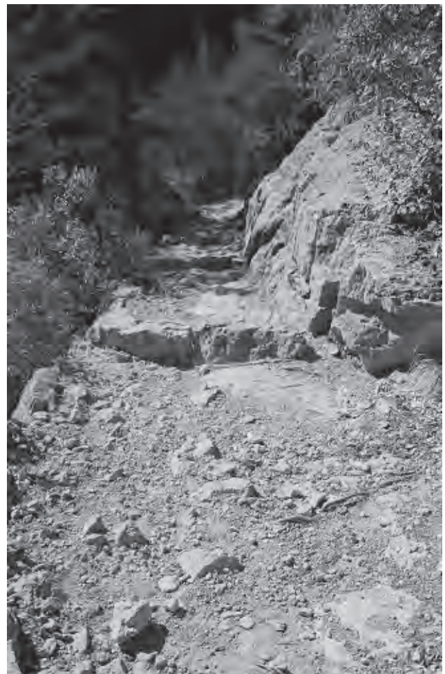
Figure 35. Portions of Ed Riggs trail are cut from rock slope; others are built up with retaining walls. Jackhammer drill marks are visible on the right slope, 2003.
