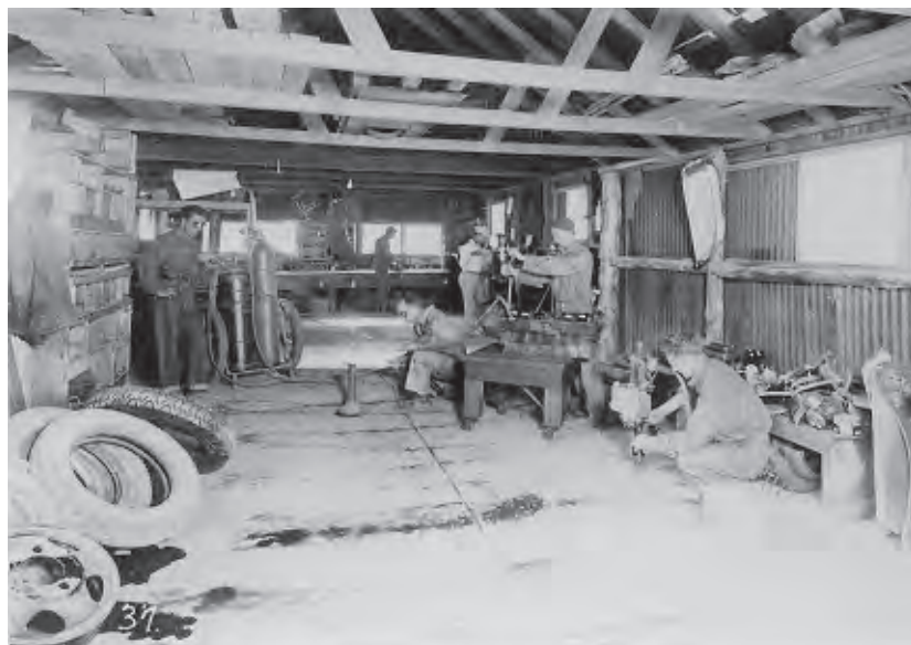
Figure 98. Interior of truck garage in National Park Service area at CCC Campsite.
