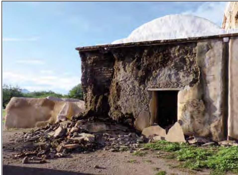
Figure 3.1. The sacristy north wall exterior of the Tumacácori Mission church (Tumacácori National Historical Park) collapsed in 2010 after a series of heavy rainfall events. (Moss 2010:12)
