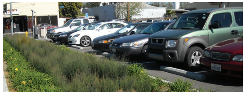
This vegetated swale in Oakland, California was retrofitted within an existing parking lot. -San Mateo Countywide Water Pollution Prevention Program 2010. pg155
