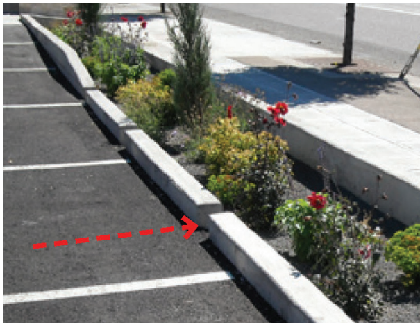
This parking lot planter uses multiple standard curb cuts to allow runoff to enter the landscape area. -San Mateo Countywide Water Pollution Prevention Program 2010. pg155
