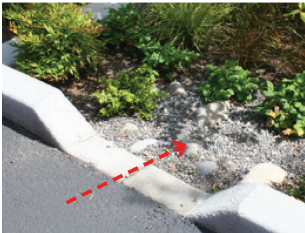
A standard curb cut allows stormwater runoff to enter a parking lot rain garden. This curb cut has 45 degree chamfered sides. -San Mateo Countywide Water Pollution Prevention Program 2010. pg152
