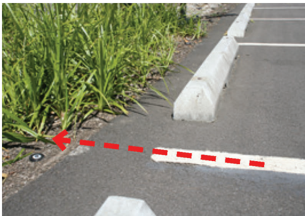
The 3 foot space in between these wheelstops allows stormwater runoff to enter a vegetated swale within a parking lot. -San Mateo Countywide Water Pollution Prevention Program 2010. pg155
