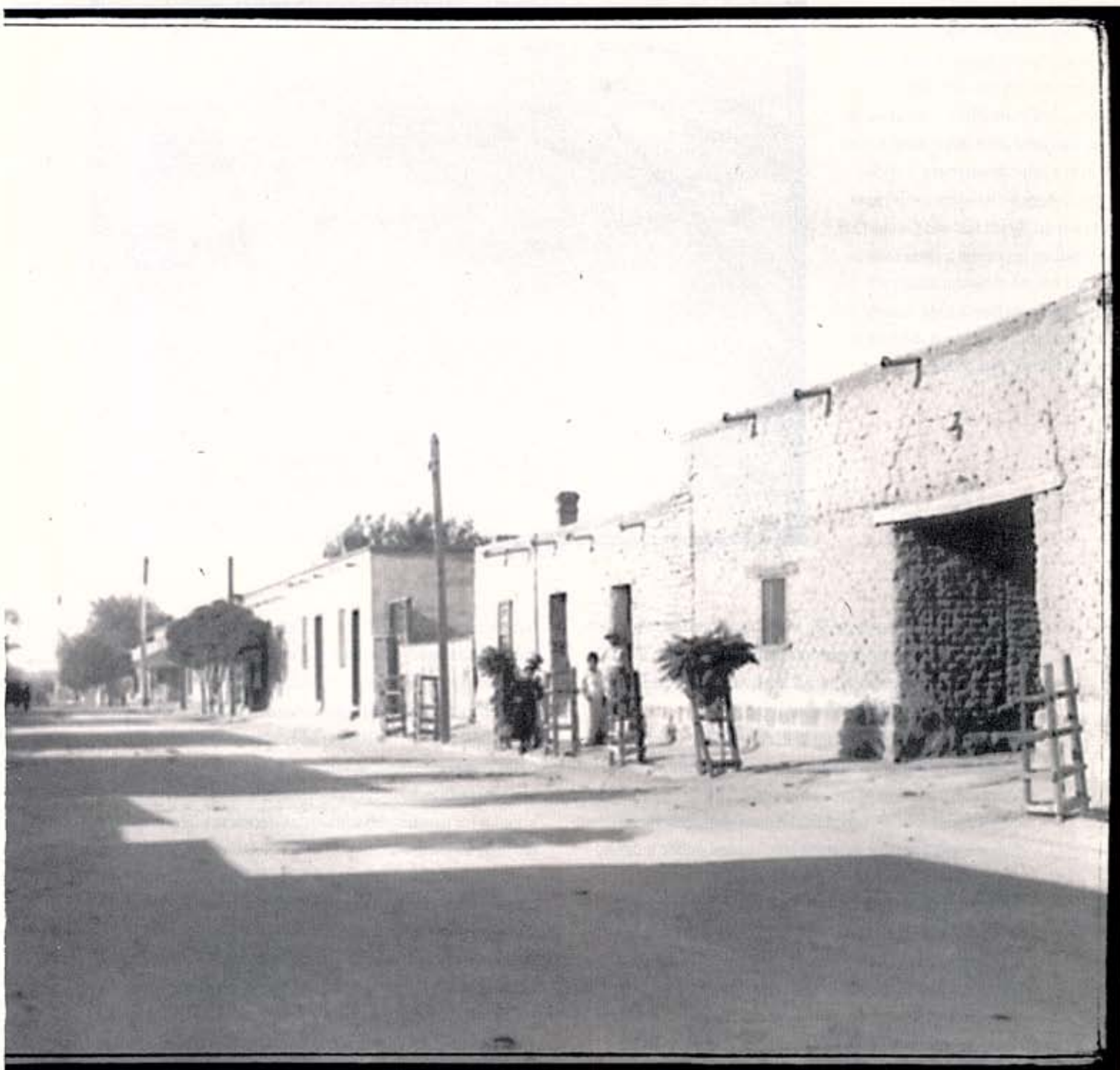
South Convent Street in the Barrio Libre Historic District, circa 1896. Tucson's Spanish and Mexican barrios, or neighborhoods, are characterized by rowhouses placed right against the street that define a perimeter around a verdant central open area. There, families and neighbors defined a sense of community through a shared common purpose that extended from security to raising domestic crops and animals. (Photograph courtesy of the Arizona Historical Society, AHS 24329)
