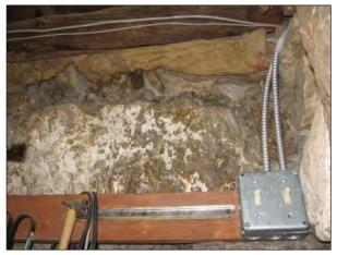
FIG. H6: North wall showing conduit. Note burlap in-fill between wall and ceiling, 2007.
