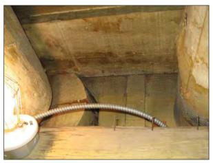
FIG. 09: Gaps between a ceiling member and the wall covered with a screen, 2007.
