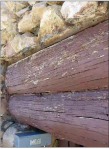
FIG. E54: Peeled paint on the lintels above the west elevation clerestory window, 2007.
