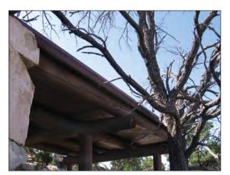
FIG. S27: Tree in contact with the porch addition roof creating a potential fire hazard, 2007.
