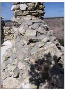
FIG. E18: Excessive and incompatible mortar applied to the Secondary Room chimney, 2007.
