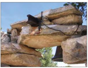
FIG. S31: Railroad track support for the bell on the corbel arch, 2007.
