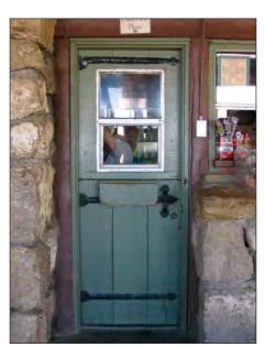
FIG. E40: Kitchen Dutch door with modern alterations including double-hung aluminum frame window and fold down shelf, 2007.
