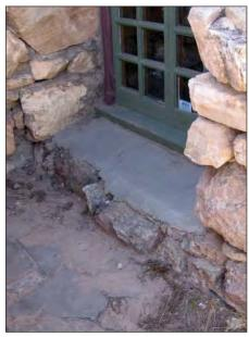
FIG. E19: Mortar applied on the stone outside of the east Secondary Room window, 2007.
