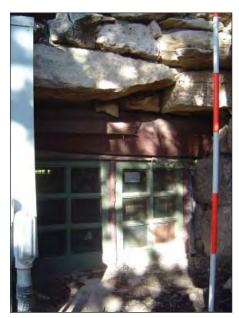
FIG. E57: Office window on west elevation. Note the duct tape and plastic applied around the window and masonite boarding in the bottom right glass pane, 2007.
