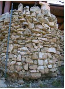
FIG. E17: Erosion at the base of the north retaining wall. Note pipe in wall. This rounded wall is presumed to cover a cistern, 2007.
