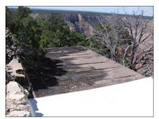
FIG. E35: View of the porch roof facing northwest showing the treatment of the historic roof in the foreground and the damaged addition roof at center, 2007.
