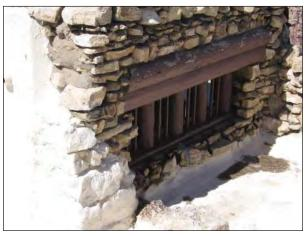
FIG. E48: East clerestory. Note the elastomeric roofing material on the stones and the peeling paint on lintels, 2007.
