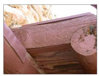
FIG. E23: Historic bark beetle damage on the porch fascia and epoxy on the log end at right, 2007.
