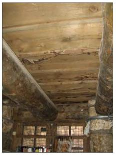
FIG. O8: View facing west showing water damage on the ceiling and wire over the windows, 2007.
