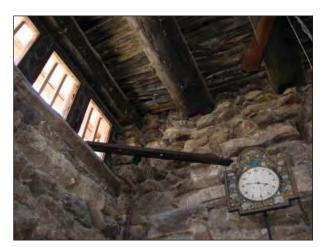
FIG. GR7: View of the southeast corner of the Great Room showing the stone walls, wood ceiling and windows, painted clock and steel c-channel for the removed propane heater. Note conduit in corner, 2007.
