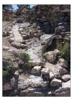
FIG. E52: Improper drainage channels to the east of the building, 2007.
