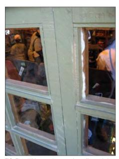
FIG. E51: White putty between the mullion and glass on the east elevation Secondary Room window, 2007.
