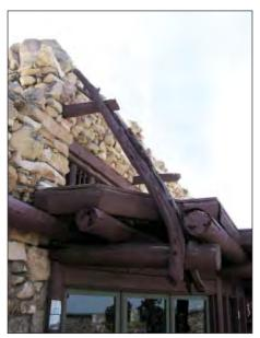
FIG. E24: Faux-structural detail at the east side of the porch roof, 2007.
