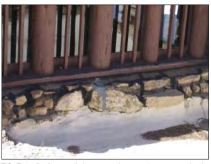
FIG. E34: Roof tar applied as mortar between the stones under the clerestory windows, 2007.
