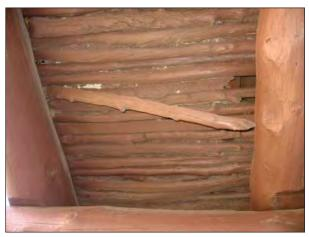
FIG. E21: Displaced latilla revealing boards on the underside of the historic porch roof, 2007.
