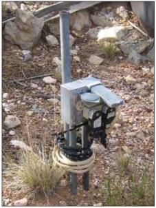
FIG. S24: Potentially hazardous outlet at the septic tank, 2007.
