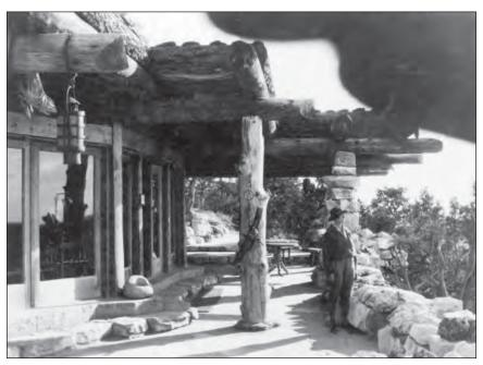
FIG. CD3: Porch area facing west. Note two steps in porch floor, projecting horizontal log beams, and concrete footing for log post, circa 1920-1930 (Source: Northern Arizona University, Cline Library, Mrs. Carl Springer Collection, NAPHS.PH.670.34).
