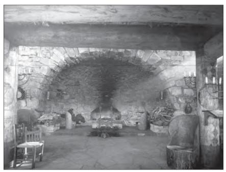
FIG. CD8: View of the Great Room facing south. Note beams and latilla of original ceiling configuration near entrance, circa 1916 (GRCA 22664).
