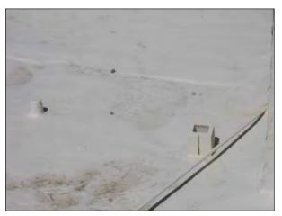
FIG. E33: View of the roof showing the concrete block and unsecured propane pipe, 2007.
