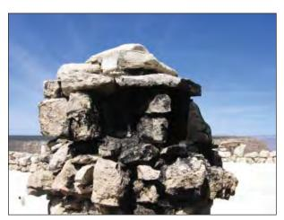
FIG. E11: View of the Great Room chimney facing north showing blocked exhaust holes, 2007.
