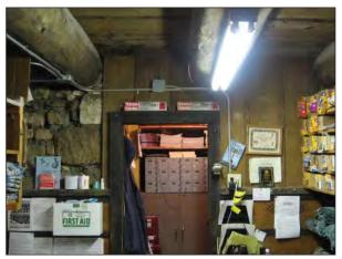
FIG. O1: View facing east showing the wainscoting over the stone wall at left and over board and batten at right. Note the missing closet door and fluorescent lighting, 2007.
