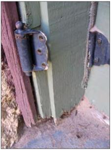
FIG. E38: Decayed door jamb and trim on the Secondary Room entrance, 2007.
