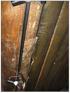
FIG. GR9: View of the modern log slab ceiling at the entrance showing the track lighting and damage caused by rodents, 2007.
