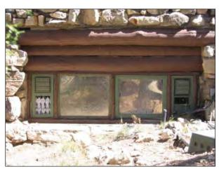
FIG. E55: Kitchen windows on the west elevation showing reflective film on center windows and vents on flanking windows. Note grey water line entering the building through the window at right, 2007.
