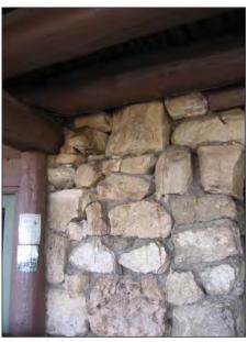
FIG. E42: Paint drip on the north elevation stone wall between the Great Room and Kitchen, 2007.
