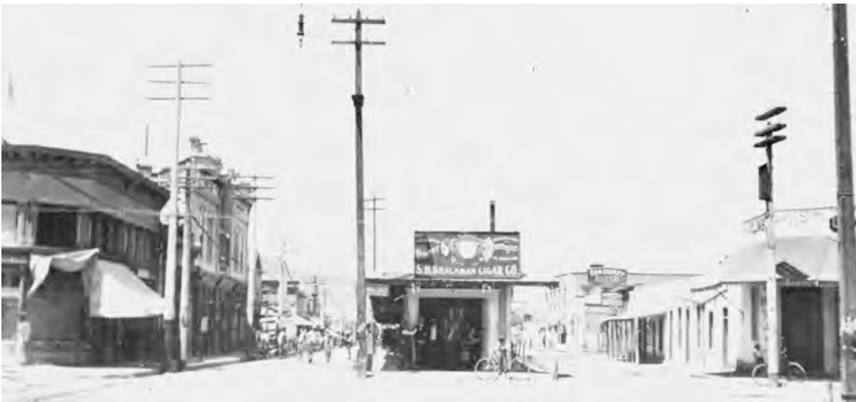
Photo 2-8. View of "The Wedge" From the East After Removal of The First Block, n.d. (from Caywood, Hooves and Rails , p. 29)
