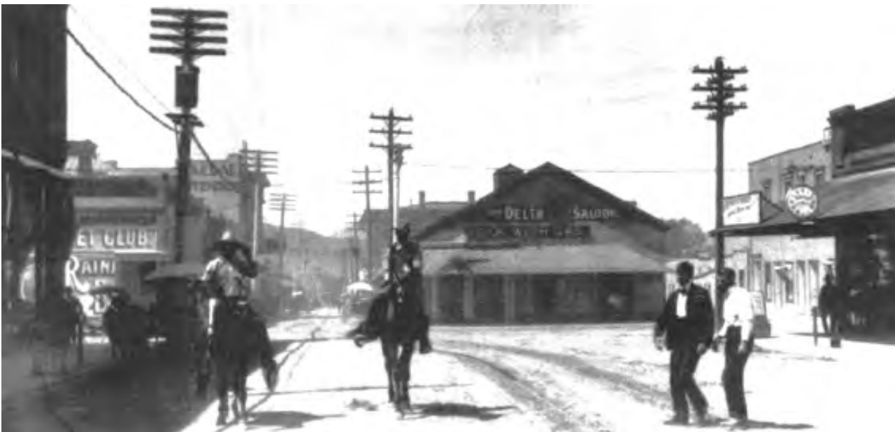
Photo 2-9. View of West Congress from the East, n.d. The remaining wedge is visible in the distance. (Arizona Historical
