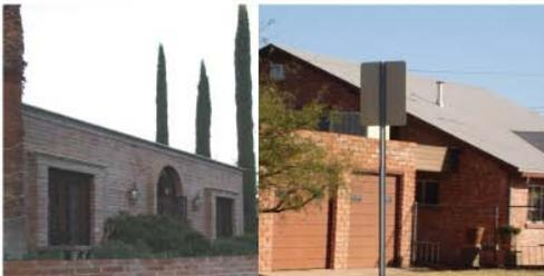
**concrete masonry units and slump block**
