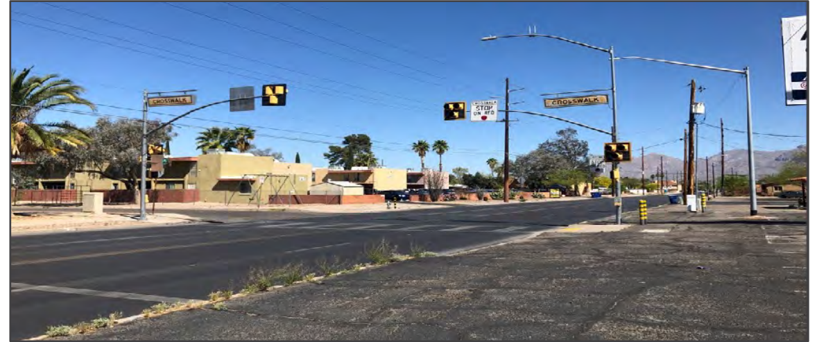
Figure 18. HAWK crosswalk at East Silver Street and North Country Club Road.
