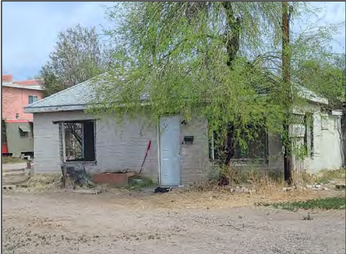
Figure 38. Derelict residence at 3139 East Bellevue Street.
