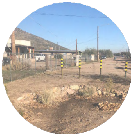
Left: An example of a Neighborhood scale stormwater harvesting basin installed in 2020 in Barrio Santa Cruz.
