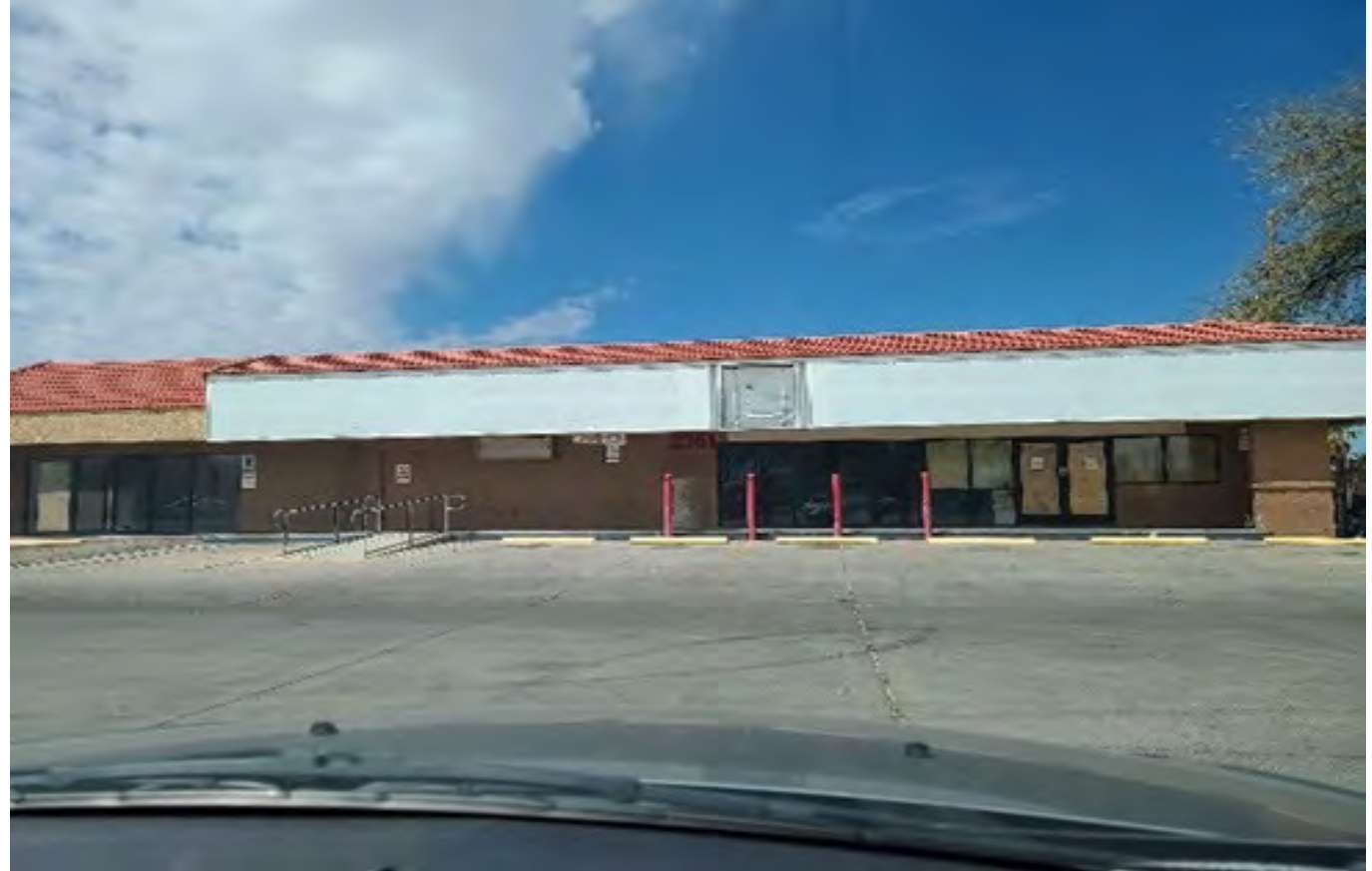
Figure 40. Redevelopment opportunity for a vacant business in Palo Verde.
