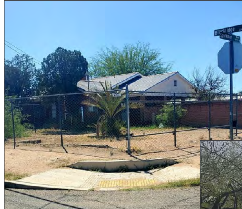
Figure 15. ADA ramp with no supportive sidewalk infrastructure.
