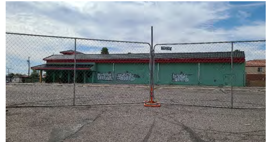
Figure 2. Redevelopment opportunity in Palo Verde.
