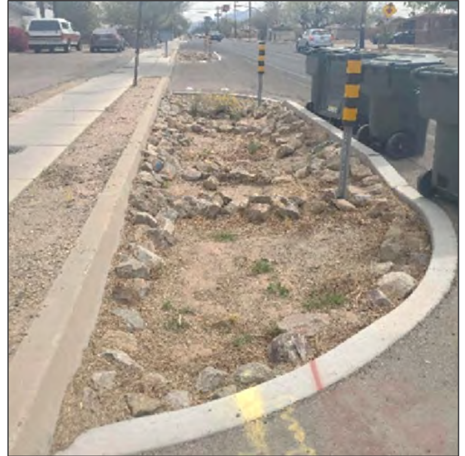
Figure 14. Poorly-maintained green infrastructure on Glenn Street.
