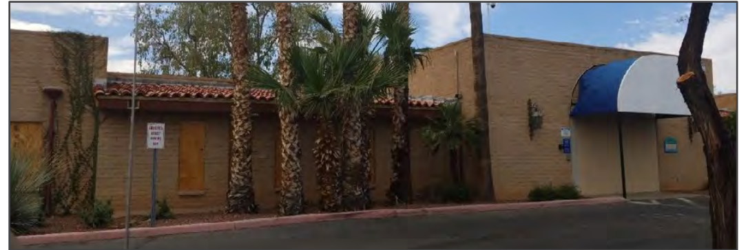
Figure 32. Vacant office building at North Haskell Drive and East Flower Street.
