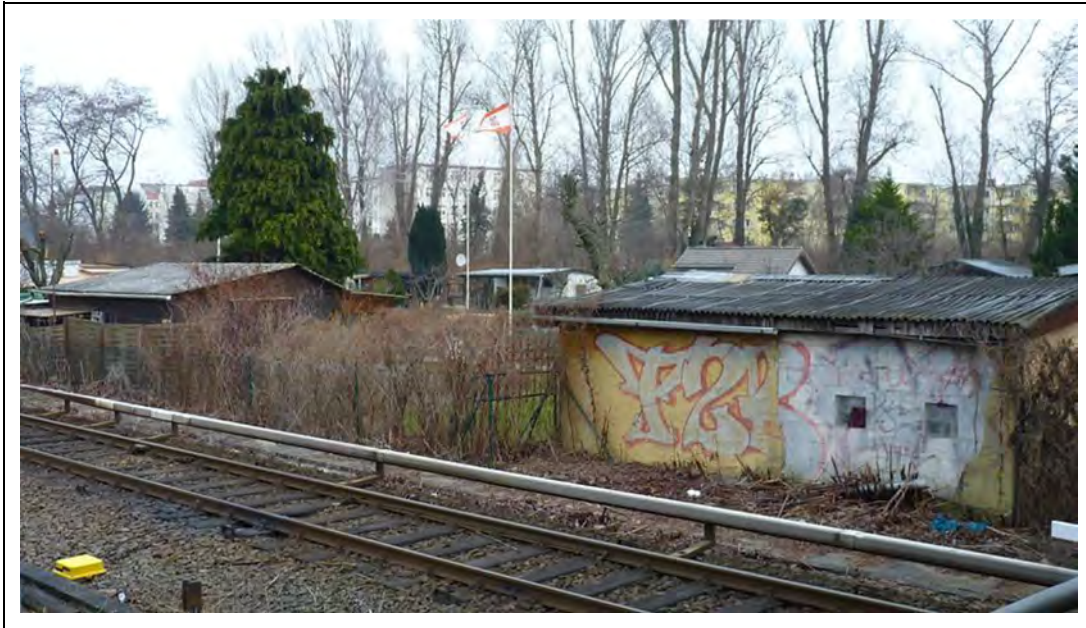
Figure 3. Sheds in community gardens used as homes. Source: "Berlin - allotments from Westkreuz UBahn" by Flickr user damian entwistle under license CC BY-NC 2.0.
