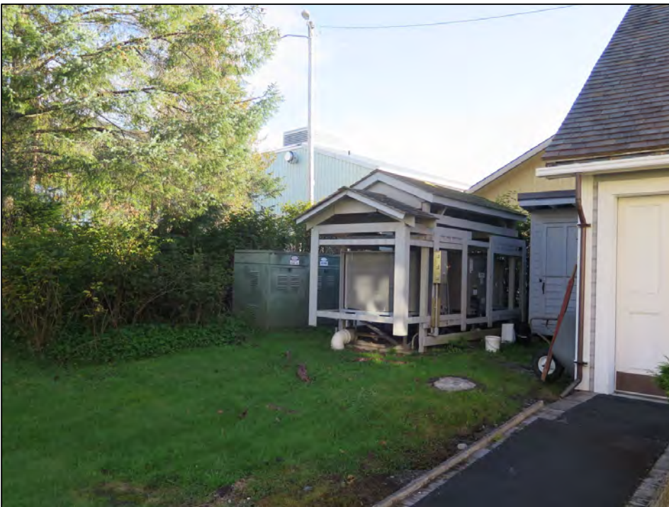
Figure 6.32. Noncontributing storage shed and utilities in the northeast corner of the Russian Bishop's House property, looking northeast, September 2016.
