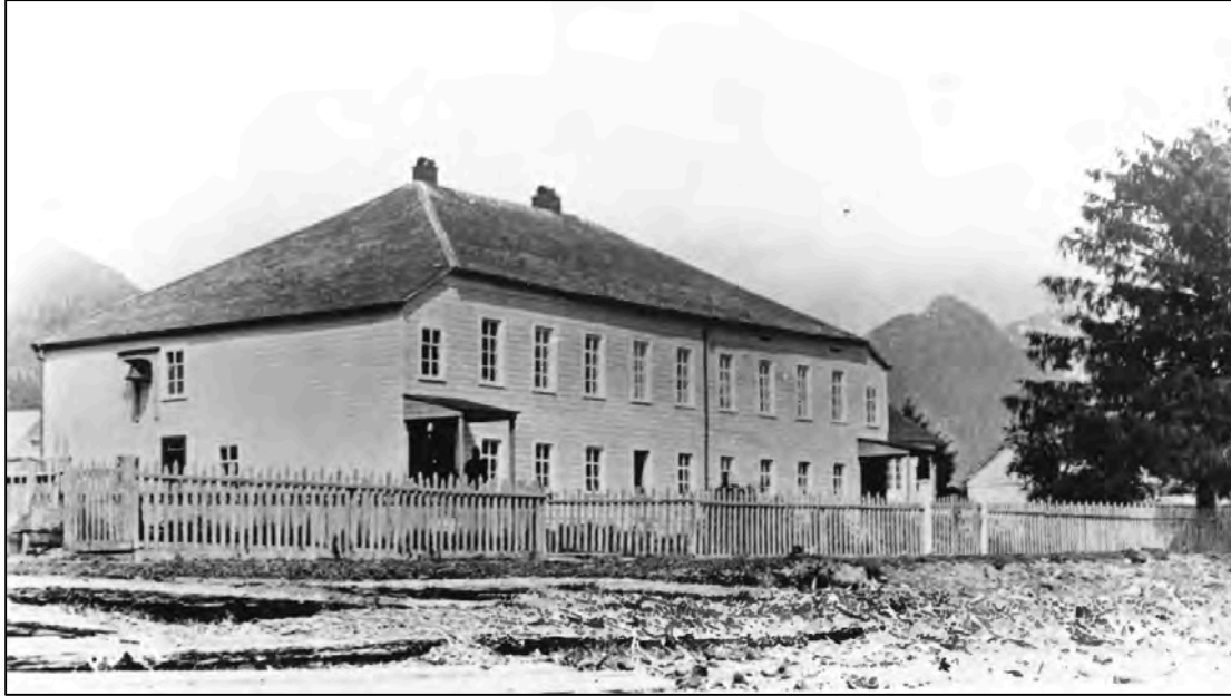
Figure 6.10. The Russian Bishop's House, looking northeast, 1890.
