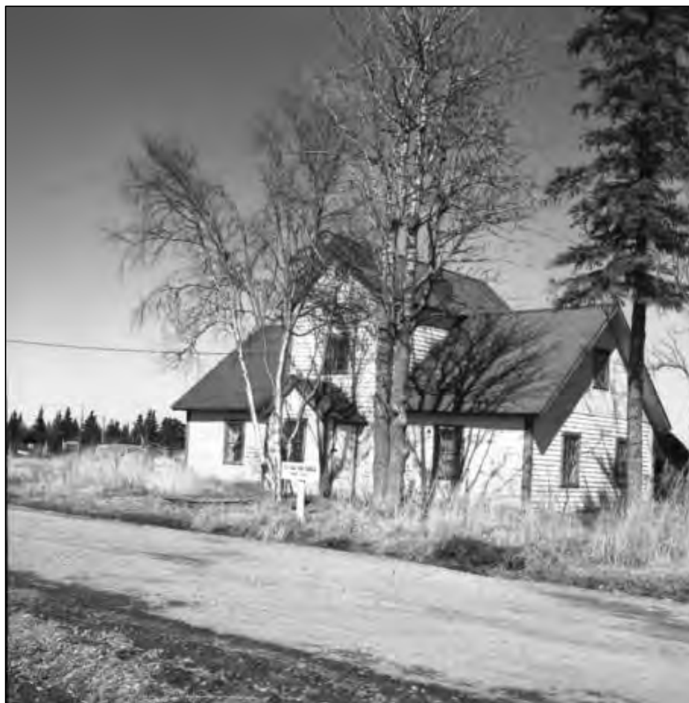
Figure 4.09.9. The rectory, looking northwest, May 2, 1963.
