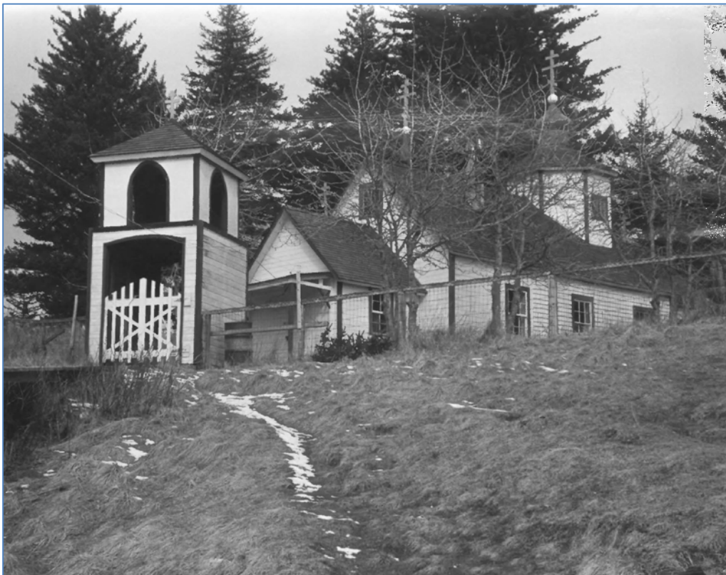
Figure 4.06.5. Church, looking uphill to northeast, ca. 1975.
