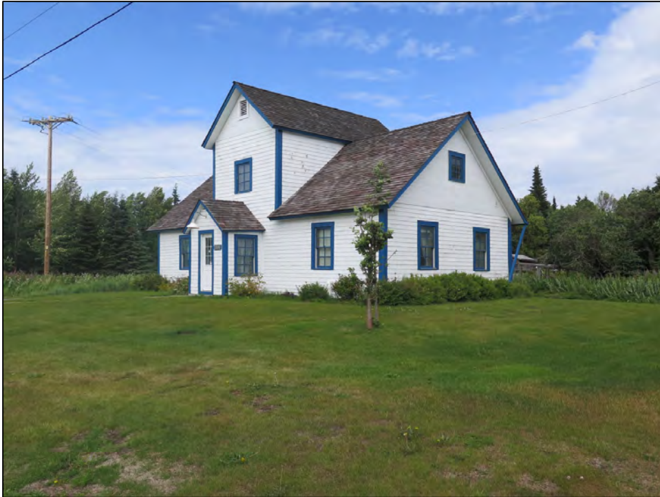
Figure 4.09.28. Rectory with overgrown road to cemetery in background, looking northwest, August 2015.
