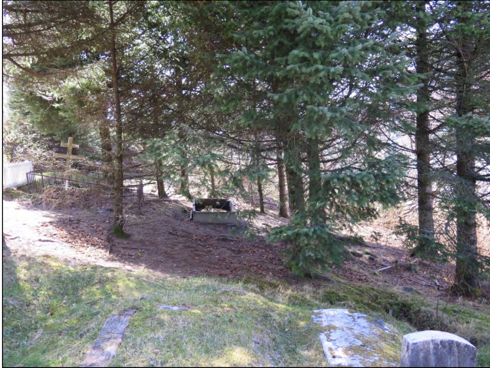
Figure 4.10. 24. Erosion of the northern slope of the new cemetery, looking west, April 2015.
