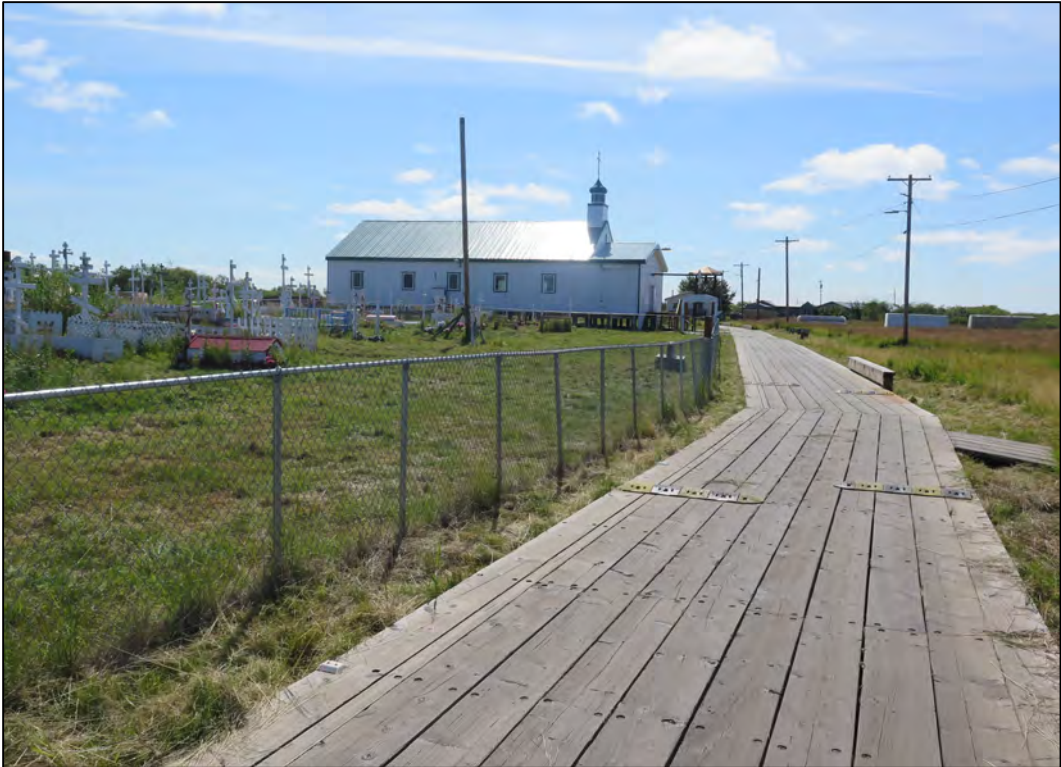
Figure 4.03. 11. Boardwalk leading to the church, looking south, August 2015.
