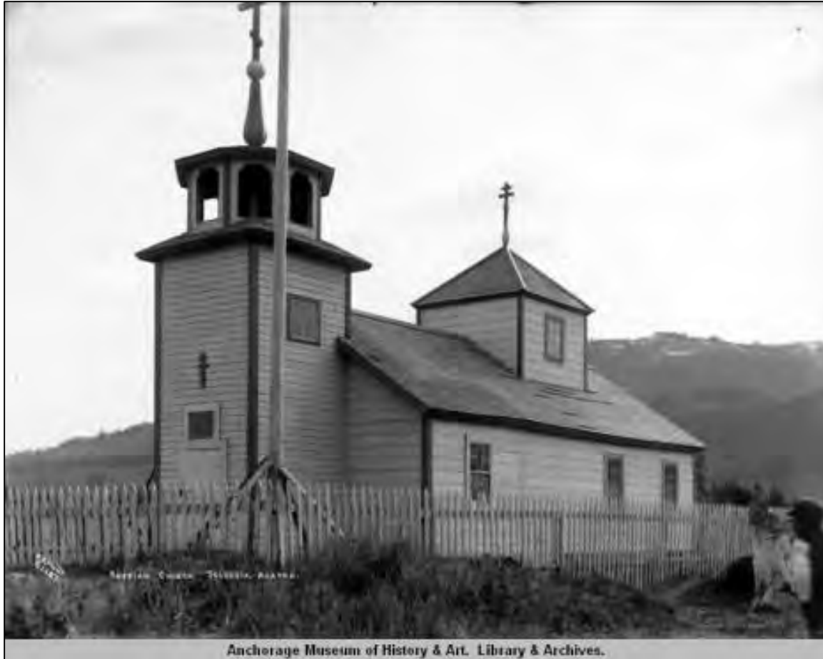
Figure 4.07. 5. Seldovia church, looking northeast, before 1913.
