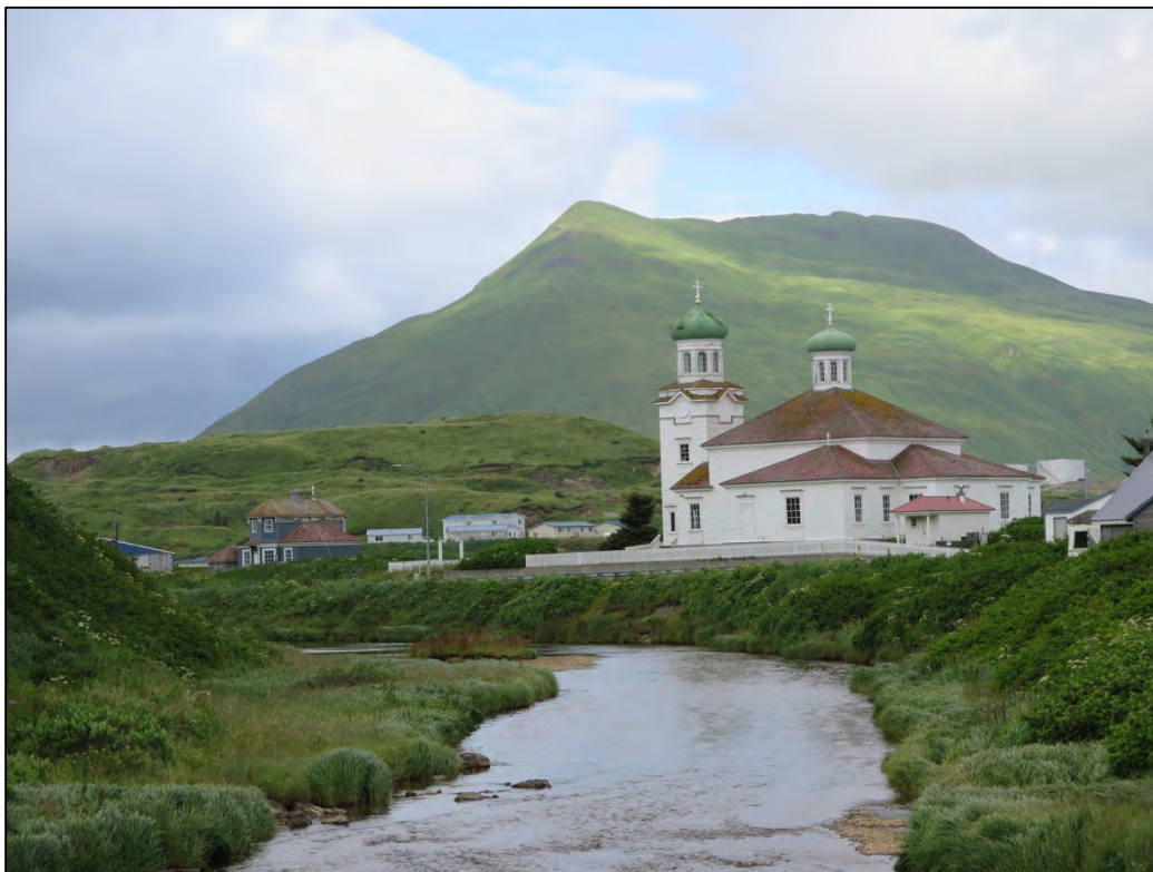
Figure 4.11. 26. View of rectory (left) and cathedral (right) with Illiliuk River in foreground, looking northwest, July 2015.
