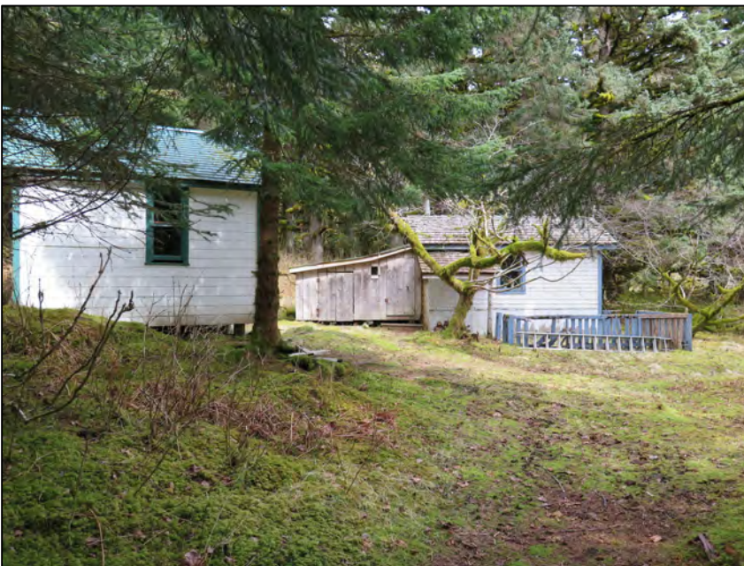
Figure 4.13.15. Fr. Gerasim's chapel (left) and cell (right), April 2015.
