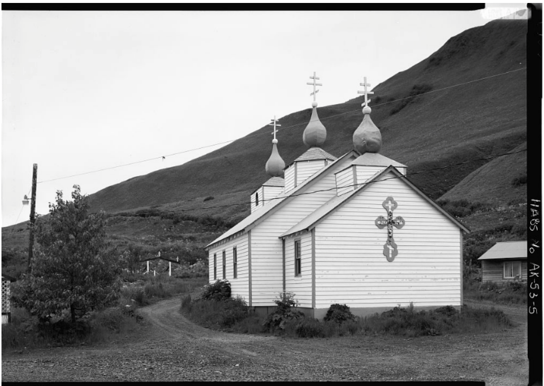
Figure 4.05. 8. East end of church, looking west, 1989.
