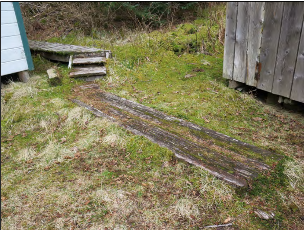
Figure 4.13.19. Boardwalk linking Fr. Gerasim's chapel and cell, April 2015.
