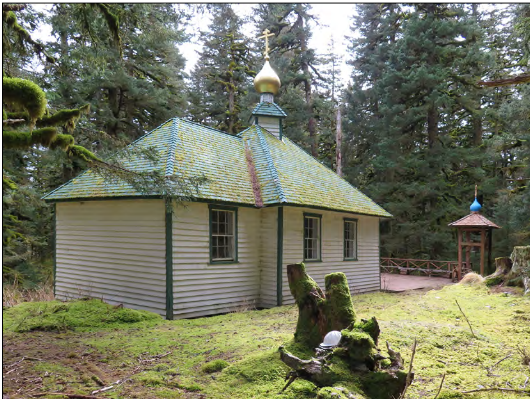
Figure 4.13.24. East end of the chapel with bell tower at right, April 2015.
