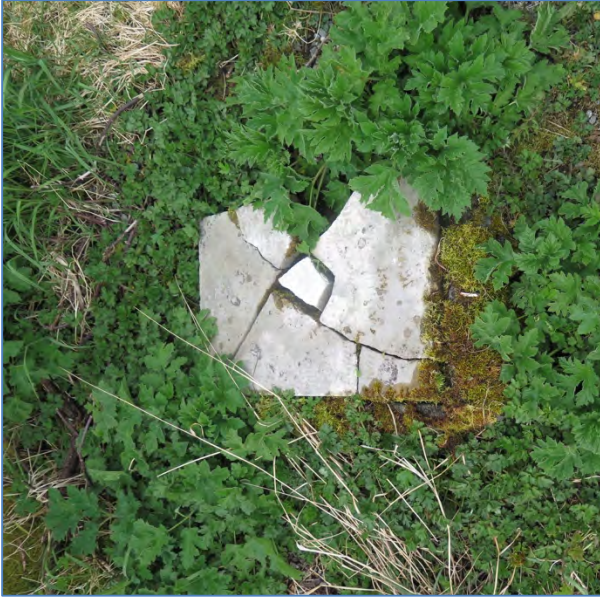
Figure 4.11.52. Damaged grave marker at Trinity Church site, looking west, April 2015.
