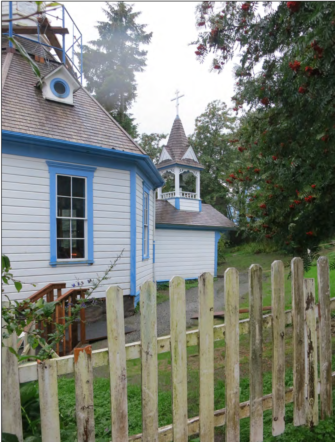
Figure 4.08.18. North side of the church and pathway leading to the entrance from the street, looking southwest, September 2014.
