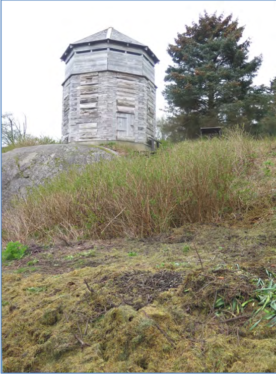
Figure 4.11.48. View of Trinity Church site, reconstructed blockhouse at upper left, looking north from Seward Street, April 2015.
