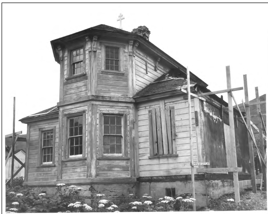
Figure 4.11. 15. Rectory after 1960 fire which destroyed the school, looking southeast, 1961.
