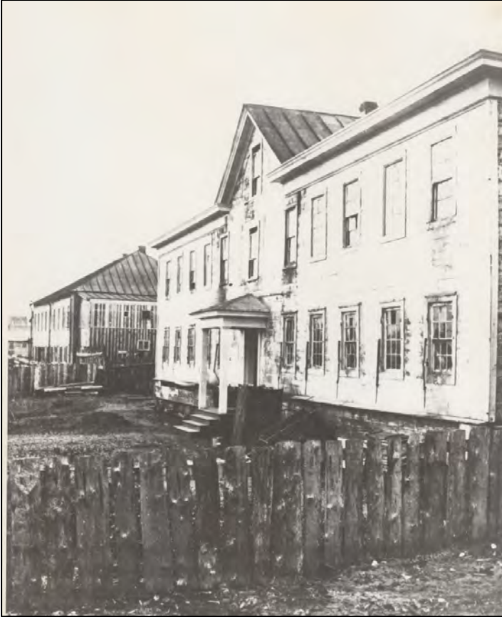
Figure 6.8. View of Seminary building in foreground with the Russian Bishop's House in the background, looking northwest, before 1882.
