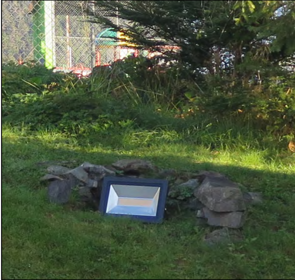
Figure 6.29. Example of lighting for the Russian Bishop's House in the northeast corner of the property, looking north, September 2016.
