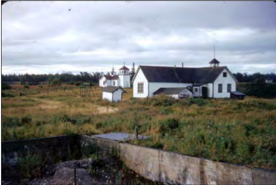
Figure 4.04.5. Foundation of parochial school, with new school and church in background, facing northwest, 1954.
