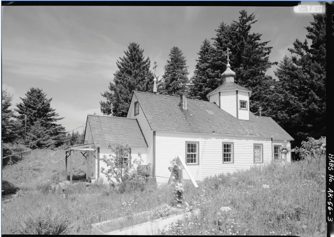
Figure 4.06.8. Church, looking northeast, 1989.
