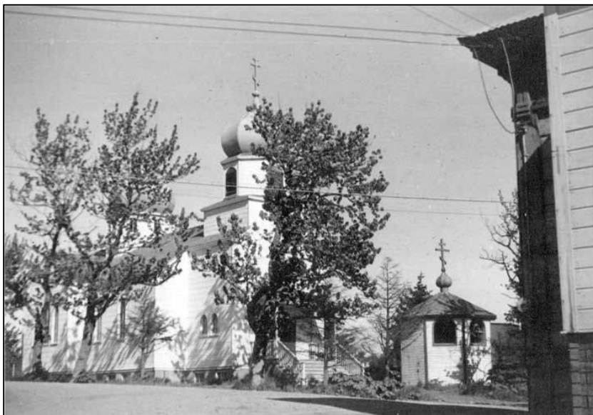
Figure 4.10. 10. Church with separate bell tower to right, looking east, after 1945.
