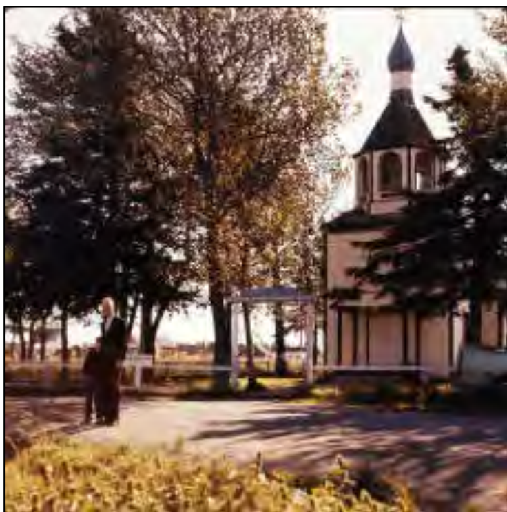
Figure 4.09.12. Kenai church, looking southwest, after 1959.
