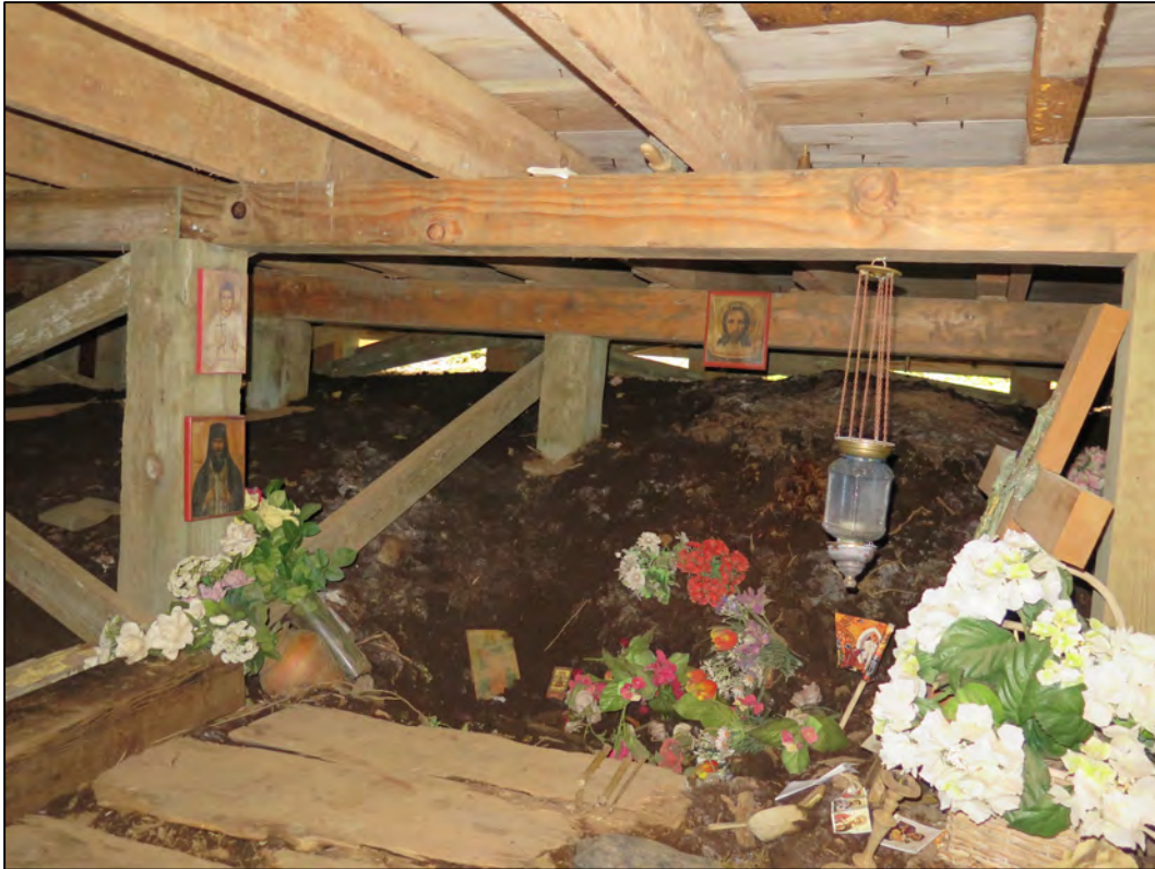
Figure 4.13.23. Crawl space under the chapel where St. Herman was buried.
