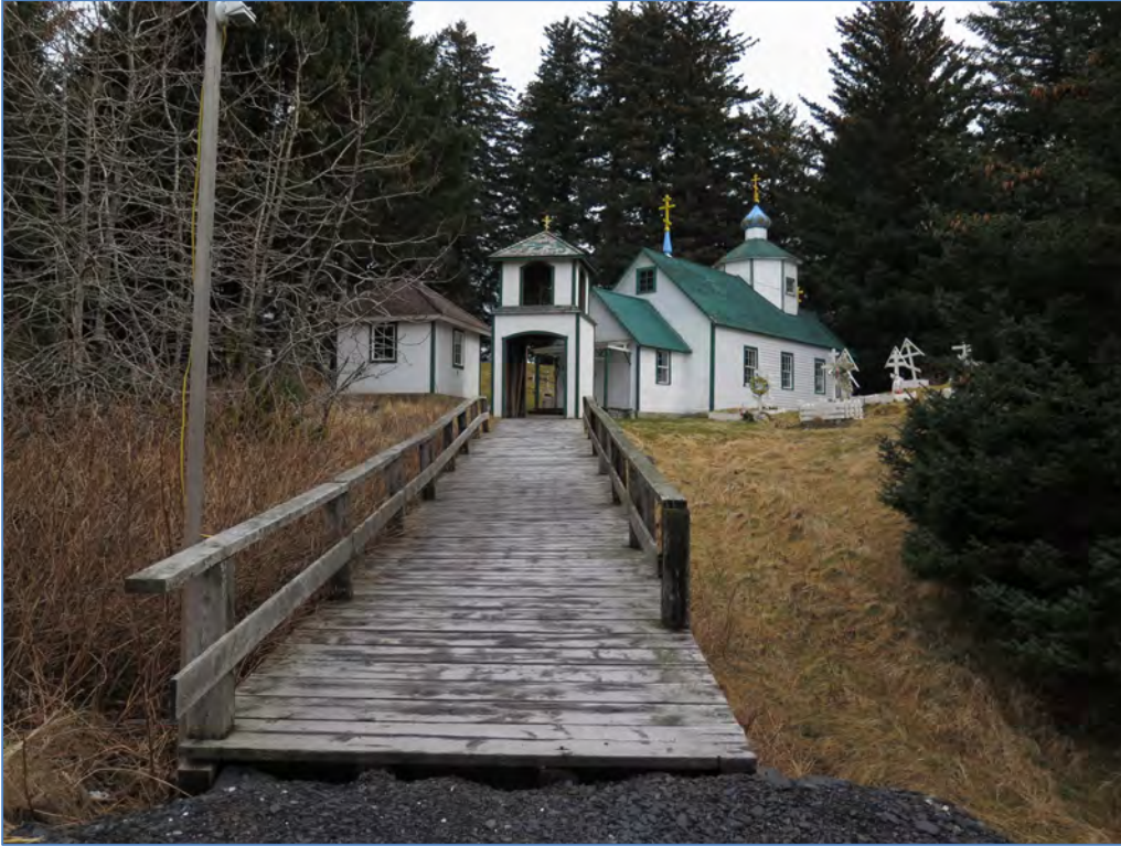
Figure 4.06.17. Bridge to the church across a drainage, looking east, April 2015.
