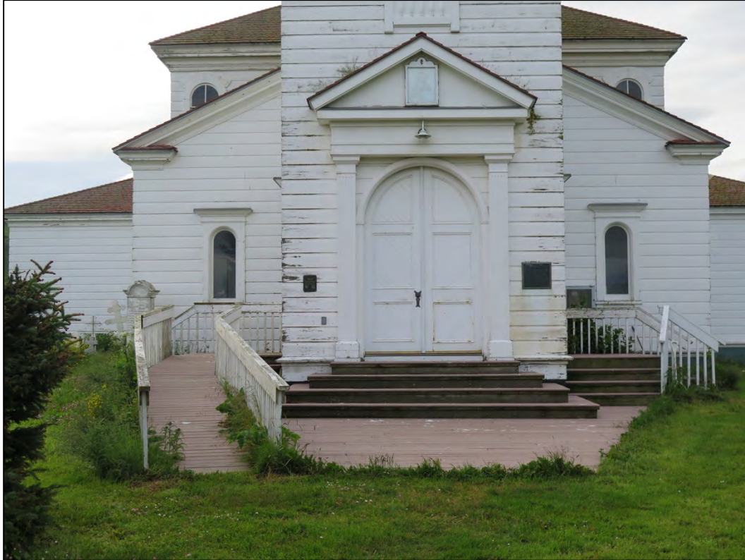
Figure 4.11. 21. West cathedral entrance with ADA ramp left and stairs right, looking east, April 2015.
