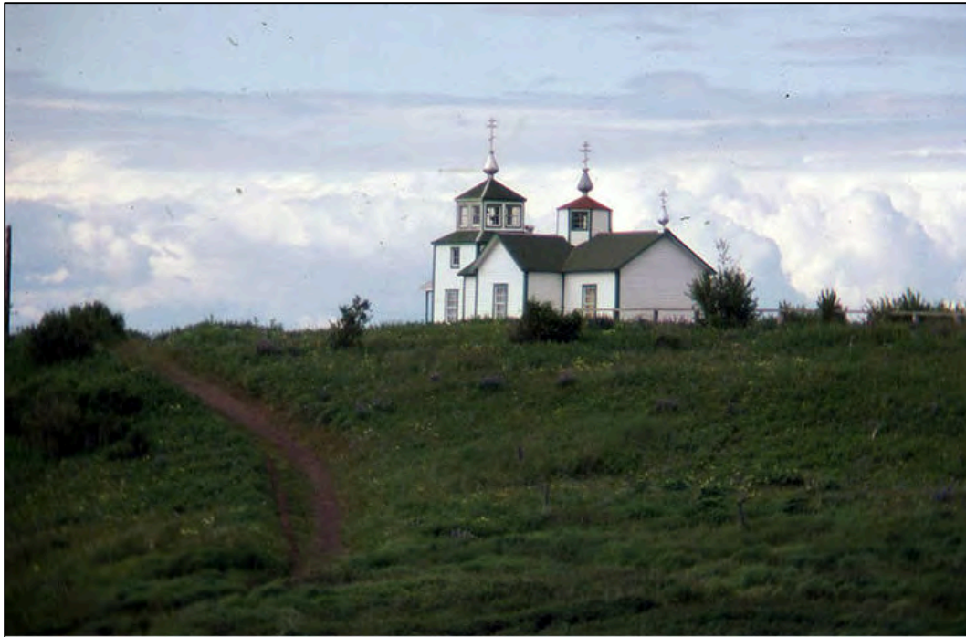
Figure 4.04.7. Ninilchik church and path leading down to the village, facing northwest, July 7, 1978.
