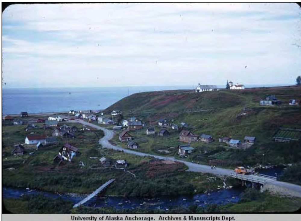
Figure 4.04.4. Village of Ninilchik church, school, and access path from across the Ninilchik River, looking northwest, 1952.
