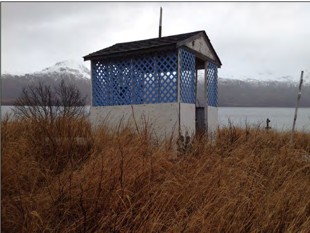
Figure 4.05. 23. Shrine of St. Basil, looking south/southeast, July 2015.
