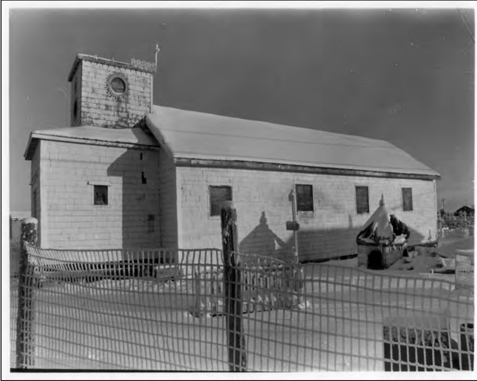
Figure 4.02. 8. Kwethluk church, looking north, 1987.
