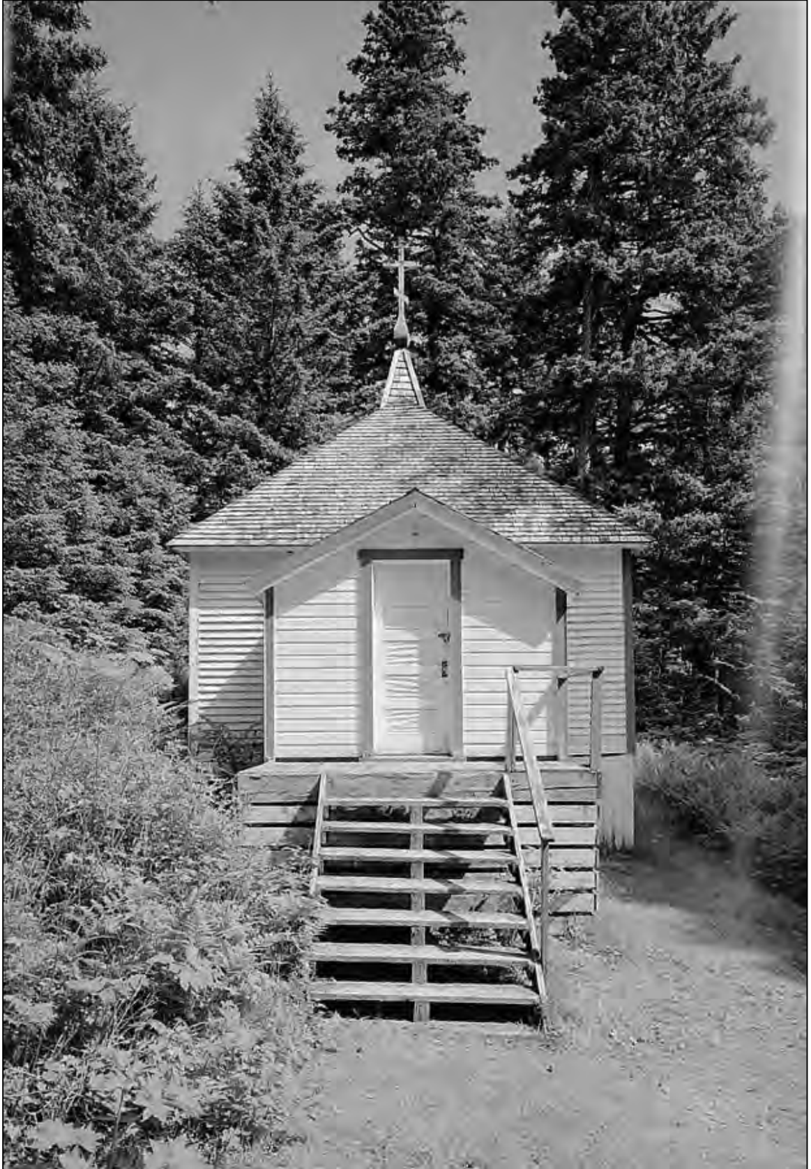
Figure 4.13.10. Chapel before 2004 renovation.
