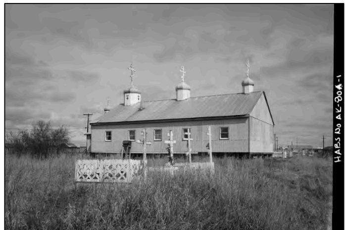
Figure 4.03. 4. New church, before the two domes to the right were removed during roof repair, looking northwest, 1990.
