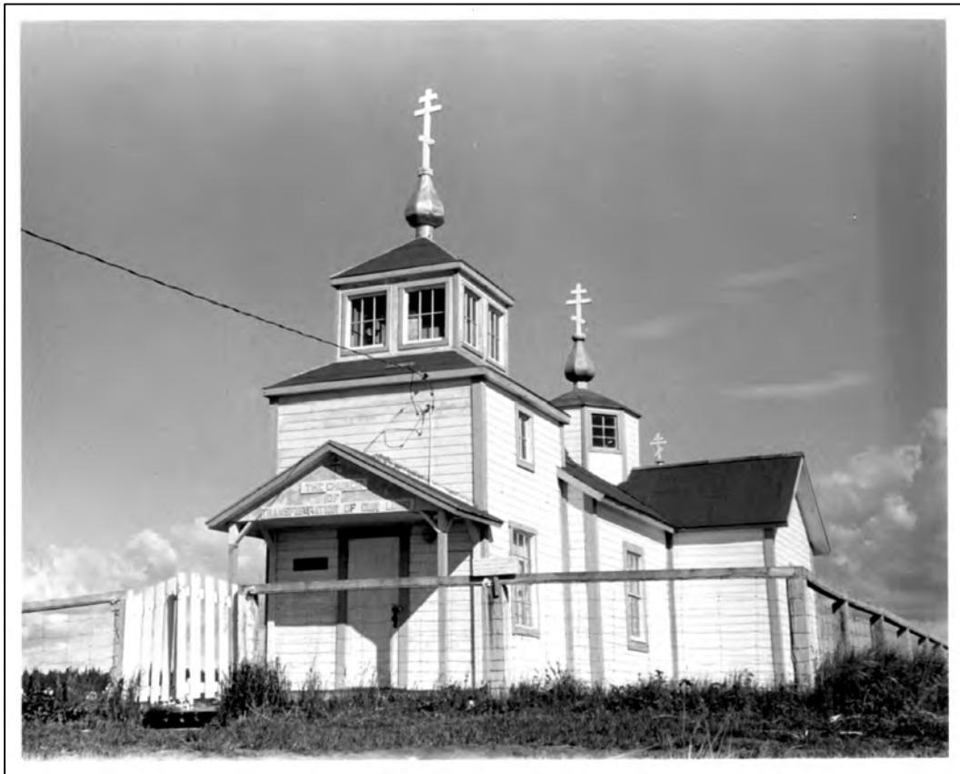
Figure 4.04.6. Entrance to church looking east/northeast, 1977.
