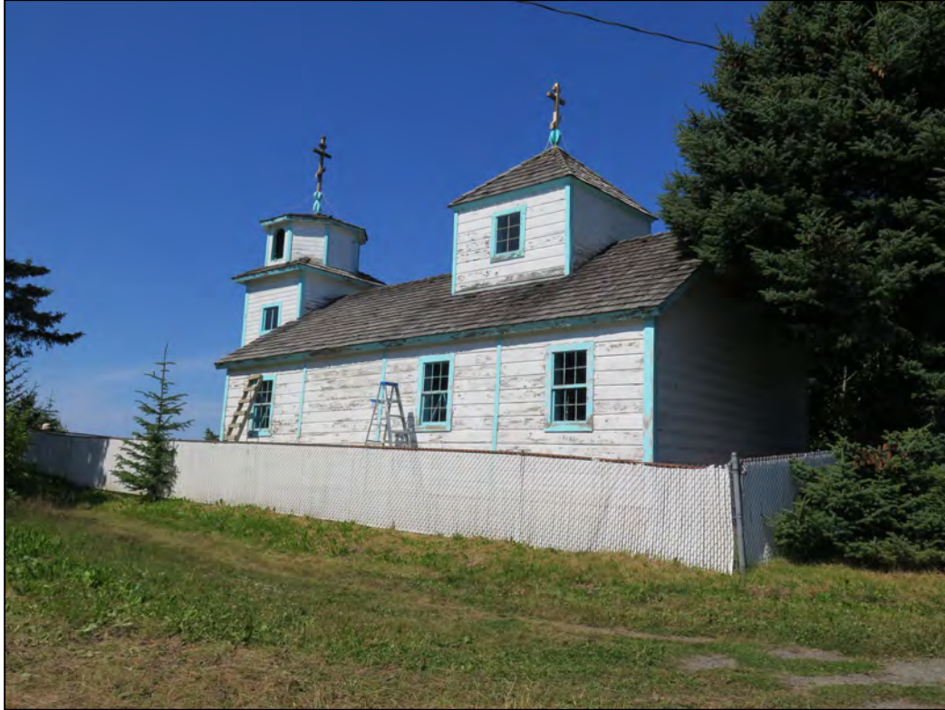
Figure 4.07. 21. Seldovia church, looking northwest, July 2015.
