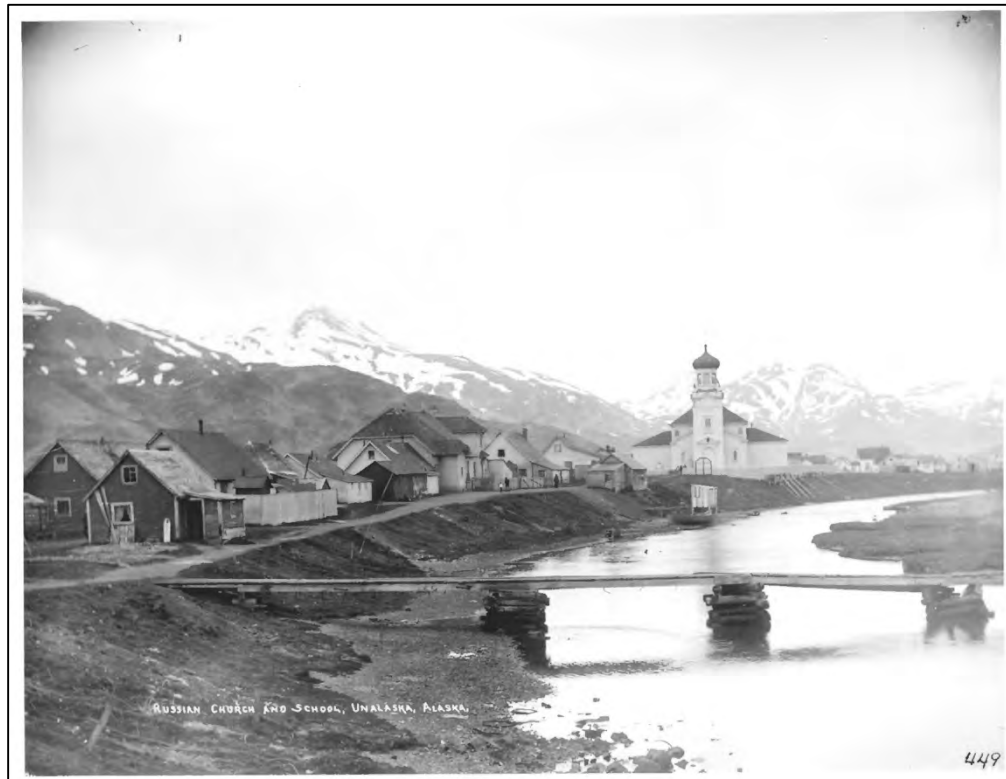
Figure 4.11. 9. Church complex, looking east, ca. 1910.
