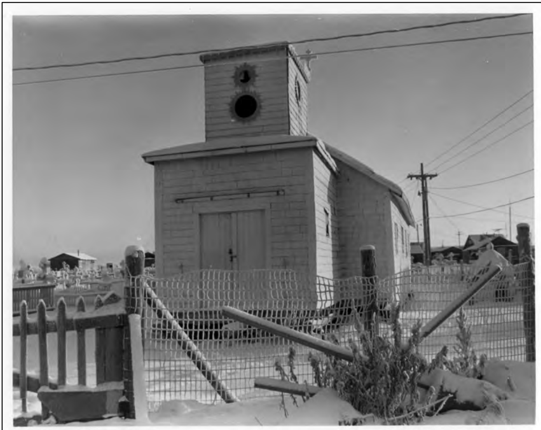
Figure 4.02. 7. Kwethluk church, looking east, 1987.
