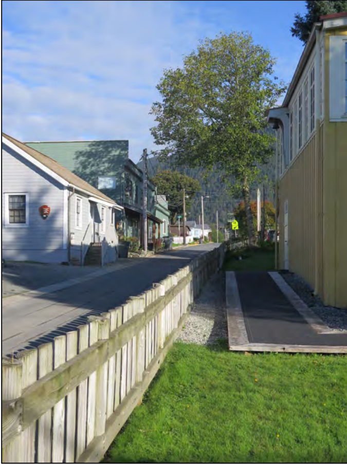
Figure 6.18. View from the west side of the Russian Bishop's House (along Monastery Street), looking north, September 2016.
