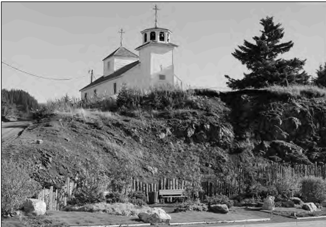
Figure 4.07. 11. Looking east from below the bluff, 1990.
