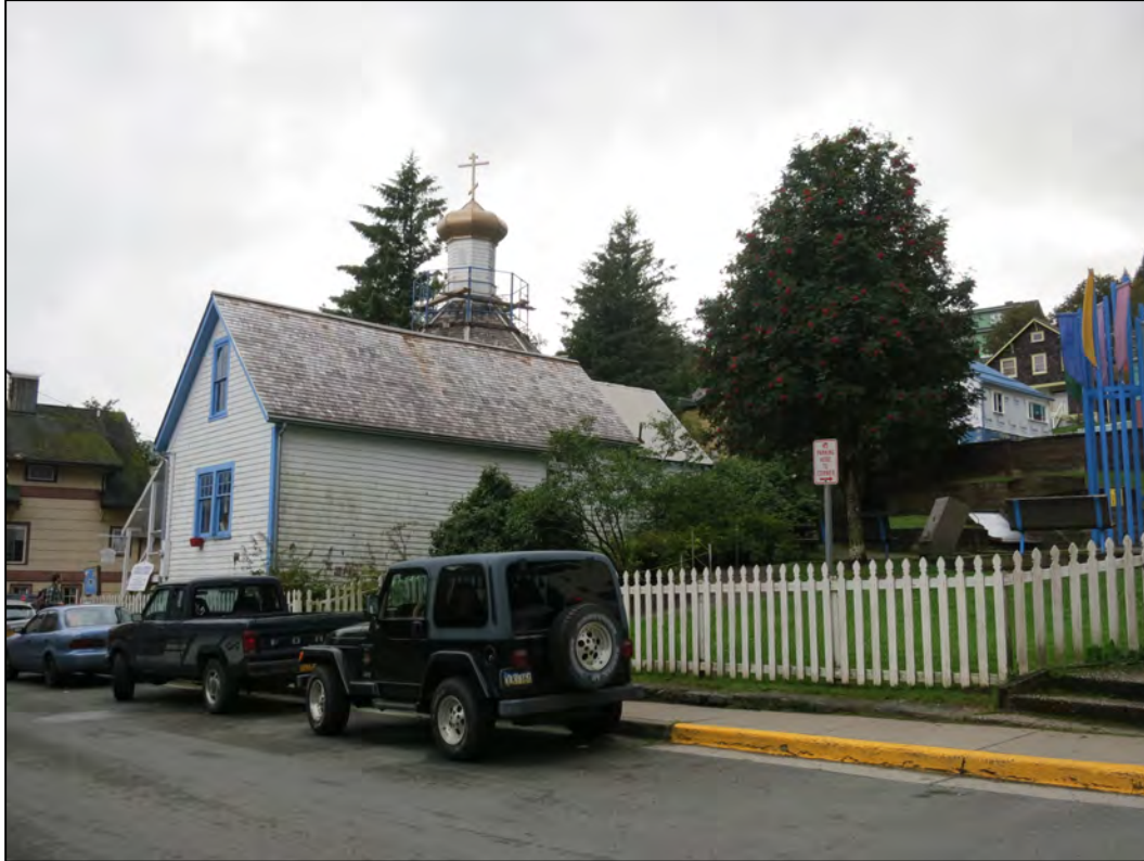
Figure 4.08.14. The rectory, looking southwest along Fifth Street, September 2014.
