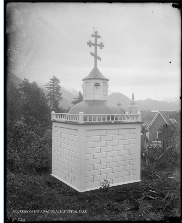
Figure 4.11.43. Shrine marking the altar location of Trinity Church, put in place by the St. Nikolai Brotherhood, looking southeast with Cathedral in background, 1907.
