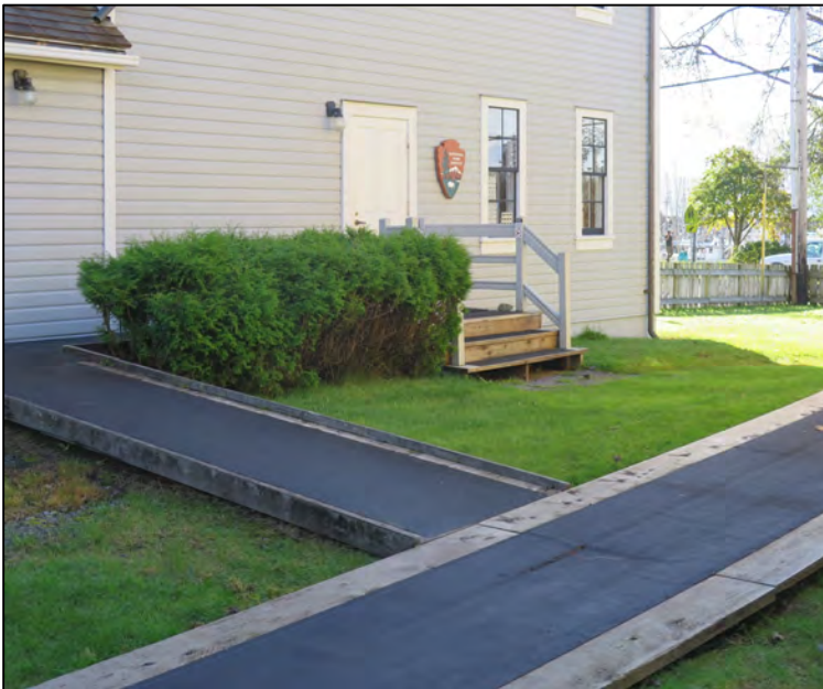
Figure 6.30. ADA access on the west side of the Schoolhouse, looking southeast, September 2016.
